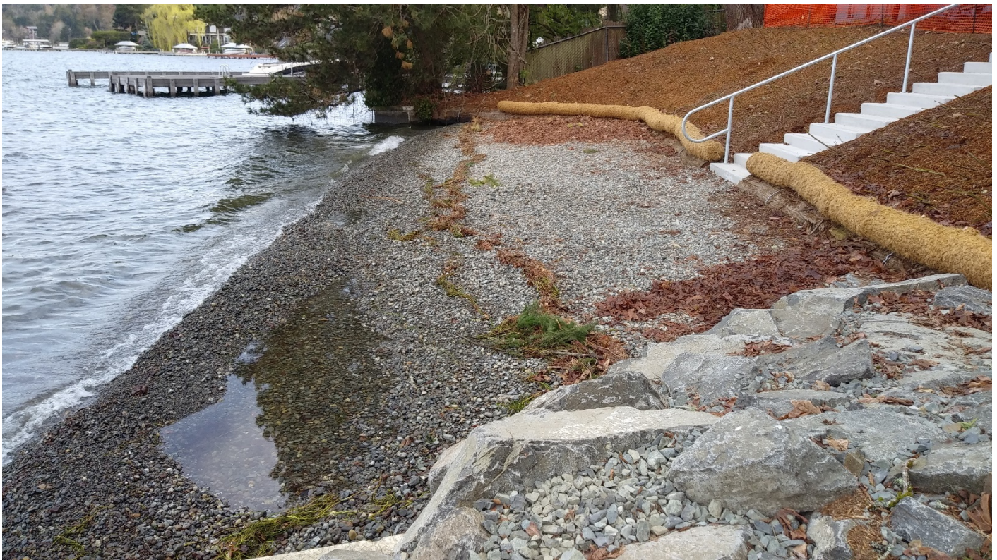
Groveland Beach looking north at the new section of shoreline restoration.
