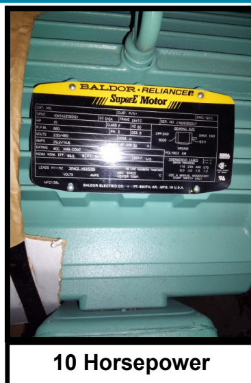
Sewer Pump Station 18 Replace 3 Cornell Pumps with 3 10 Horsepower Vaughn Chopper Pumps
