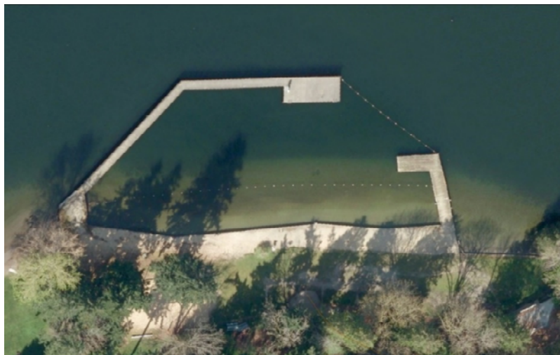
Figure 1: Groveland Beach swim area showing large dock on the left and small dock at right with the shoreline concrete bulkhead in between.
