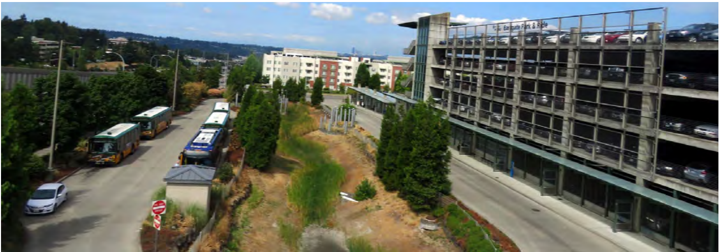
Eastgate Park-and-Ride. Source: Andy Nystrom via Flickr
