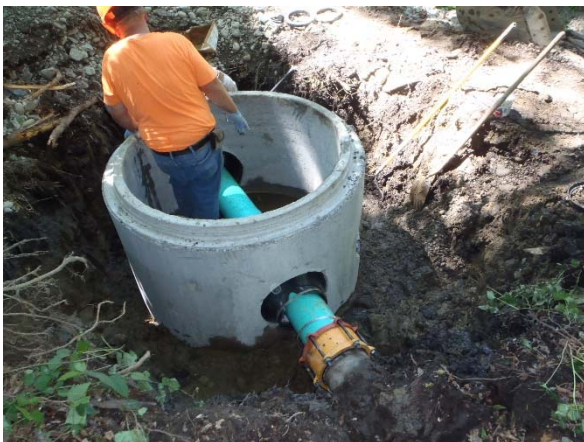
Manhole connection
