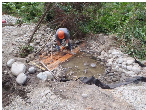
Watercourse stabilization with stream rocks and log weirs
