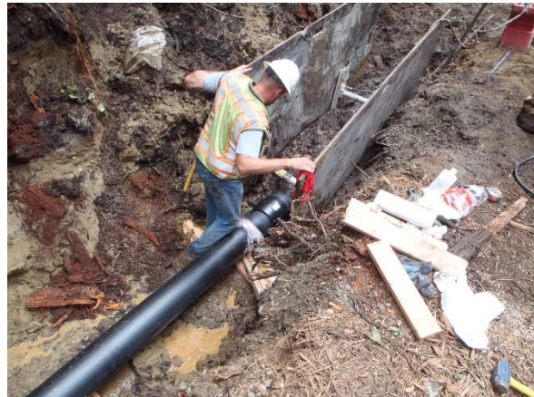
New sewer main installation
