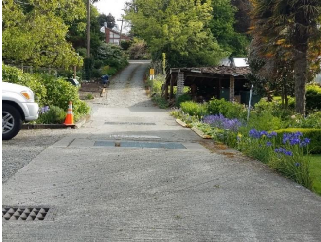
View of Freeman Avenue looking uphill east towards West Mercer Way at the top of the hill. Pavement width is approximately 15 ft. wide, ROW width is 60 ft. wide. Residential development has encroached in the entire non-paved ROW.
