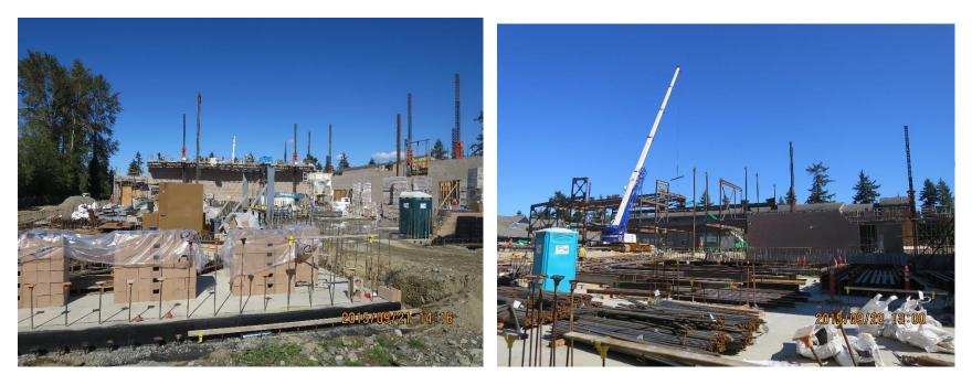
Status of Work: Approximately 30% complete Structural masonry and steel underway Completing footings at Commons/Kitchen
