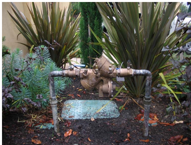
RPBA – Reduced pressure backflow assembly
