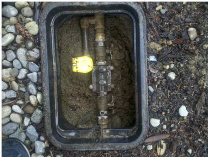
DCVA – Double check valve assembly
