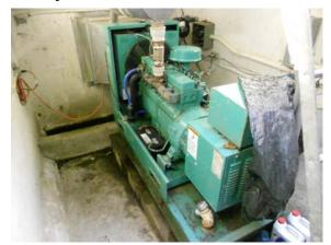
and all mechanical equipment in the station, the back-up generator that provides emergency power in the event of a power outage, and the telemetry that provides monitoring and control of the station.
