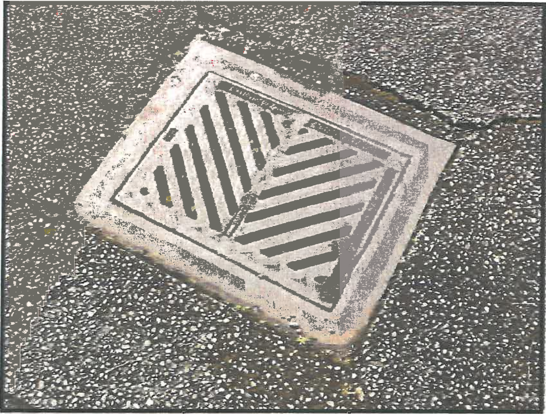
PHOTO 9: Catch basin, in driveway at 8253 SE 30 th Place, that is connected to drainage pipe.
