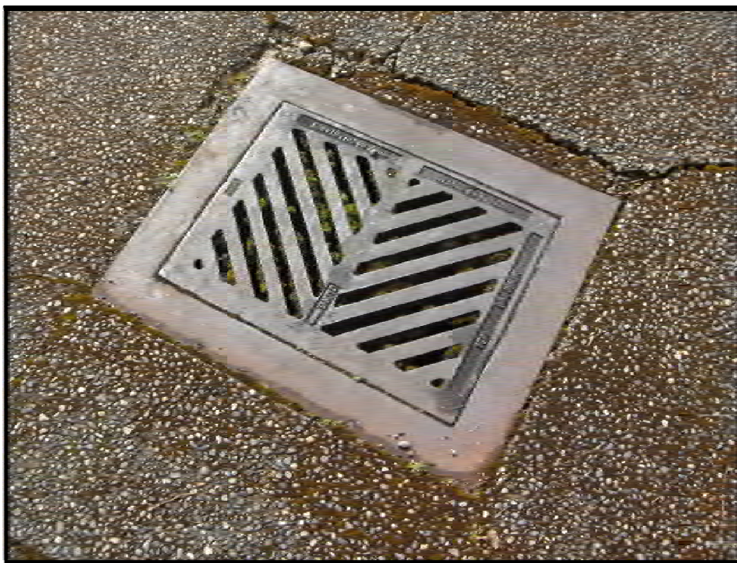
PHOTO 9: Catch basin, in driveway at 8253 SE 30 th Place, that is connected to drainage pipe.
