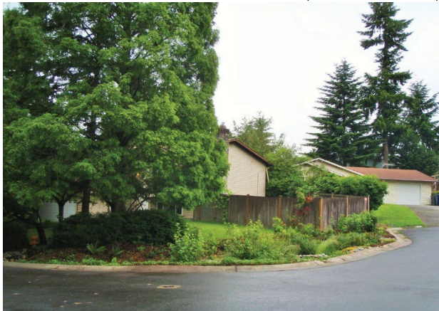
Rain garden collecting road runoff
