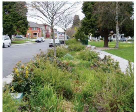
Established bioretention facility
