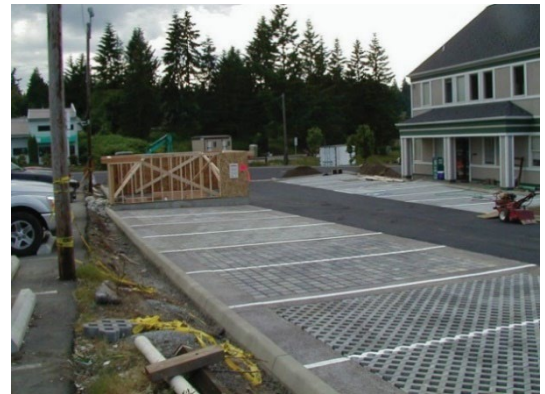
Permeable pavement installation
