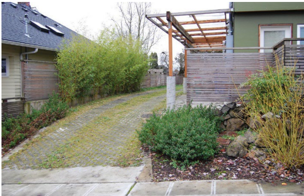
Permeable pavement driveway
