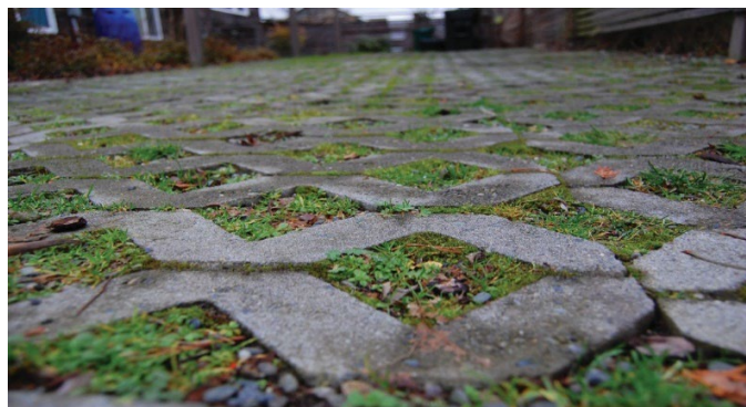
Permeable pavement driveway
