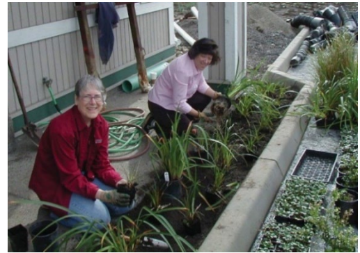
Bioretention during installation
