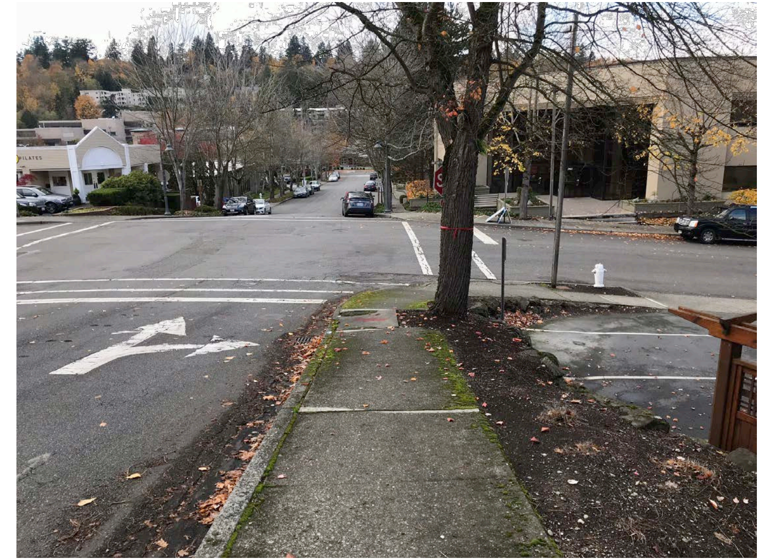
VIEW DOWN SE 30TH ST - LOOKING WEST
