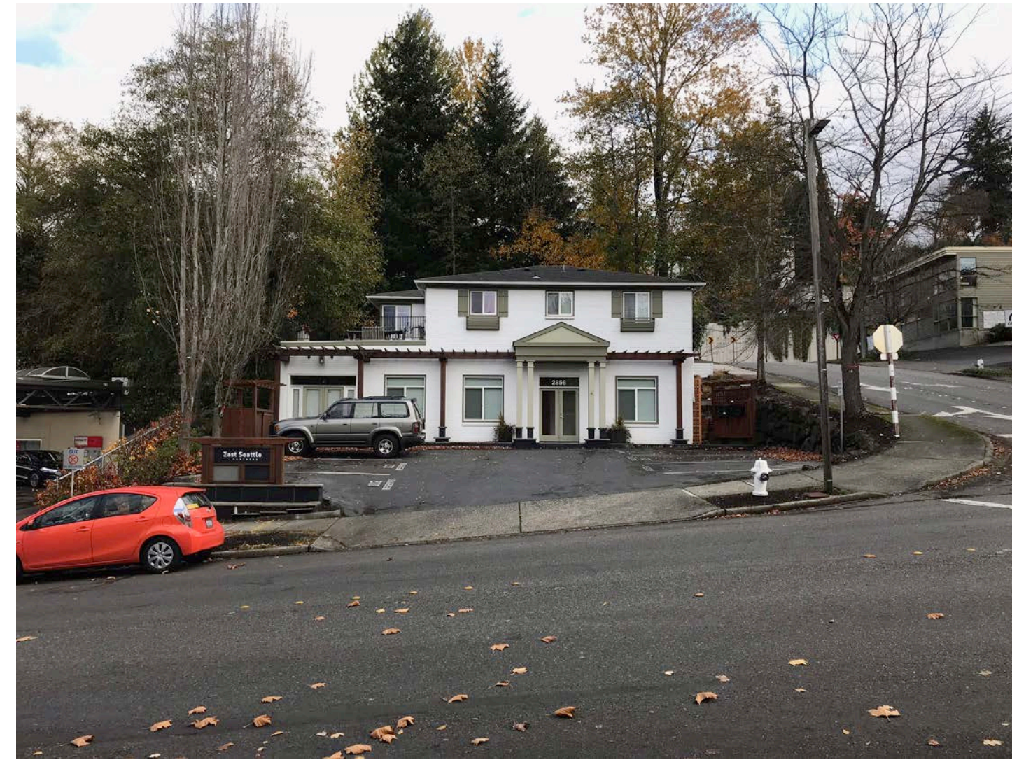
VIEW ACROSS 80TH AVE SE - LOOKING EAST
