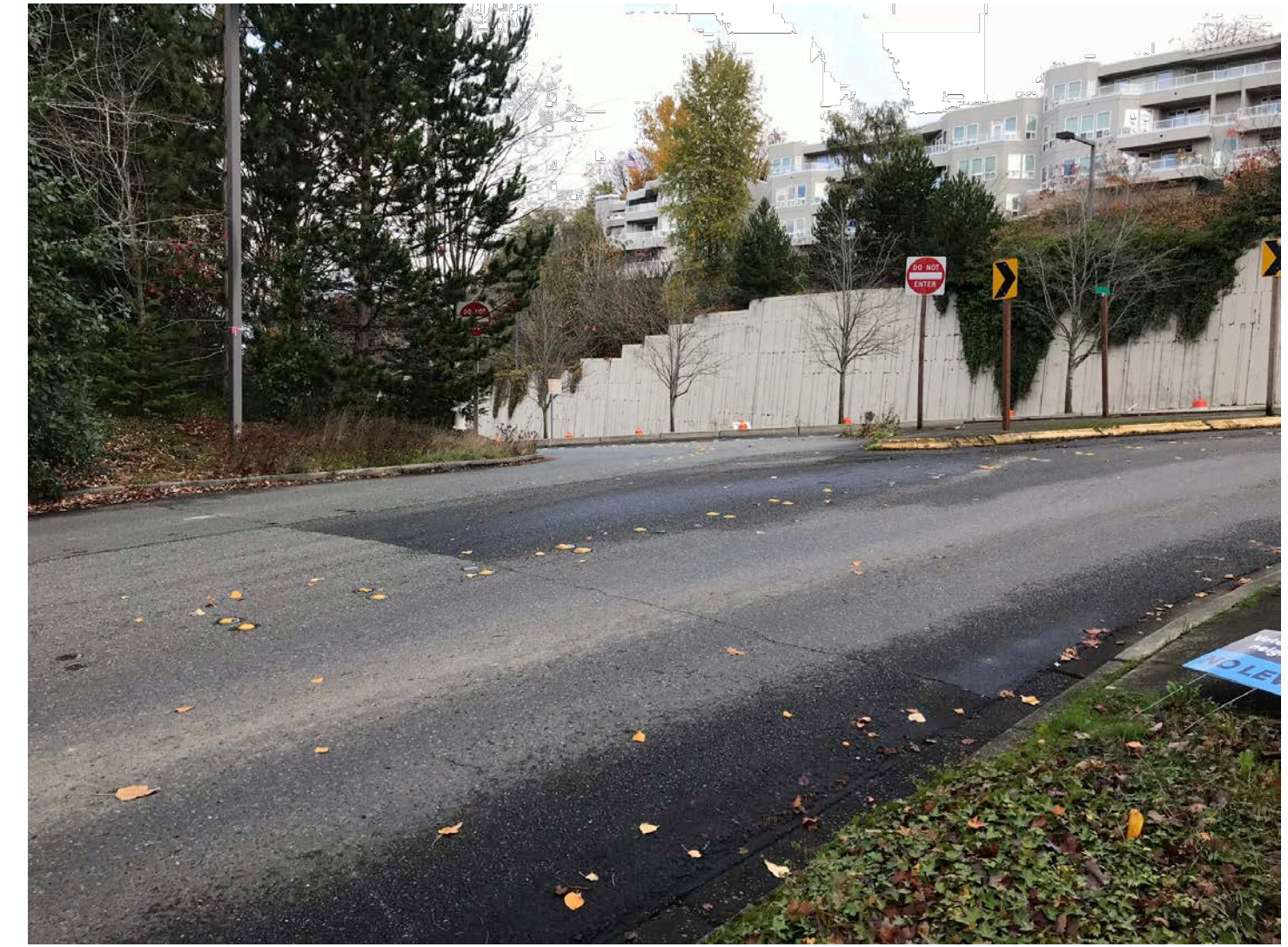
VIEW ACROSS SE 30TH ST - LOOKING EAST TOWARDS ISLAND CREST WAY
