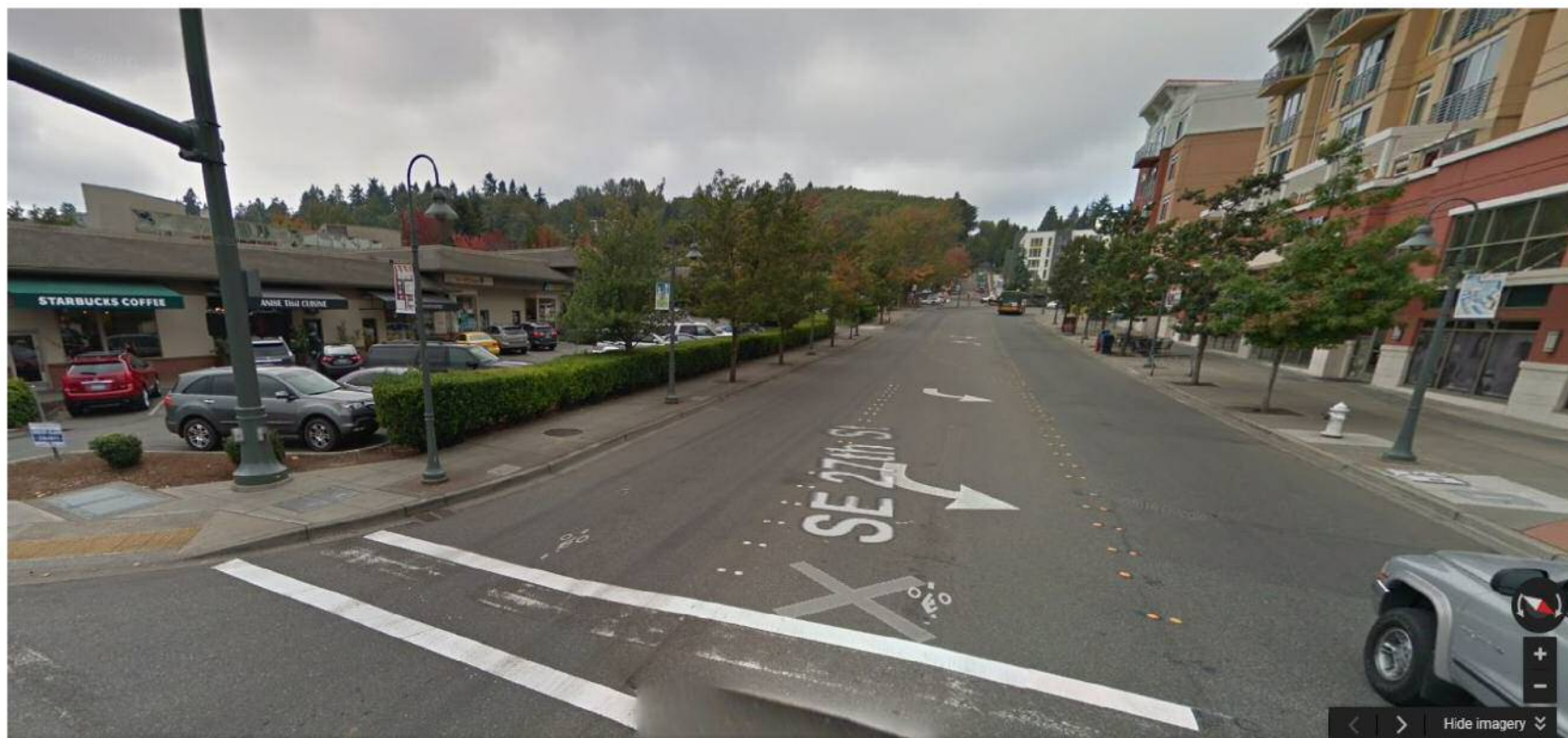
27TH STREET - WESTBOUND VIEW MERCER ISLAND, WA
