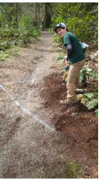
Parks staff resurfaced the north and west perimeter trails in November 2018. Over 65 tons of crushed rock was spread, graded and compacted.
