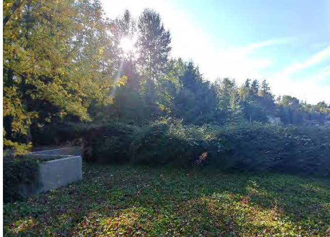
Photo 16. English ivy along bridge deck. Tree planter to the left has ample space for maintenance.
