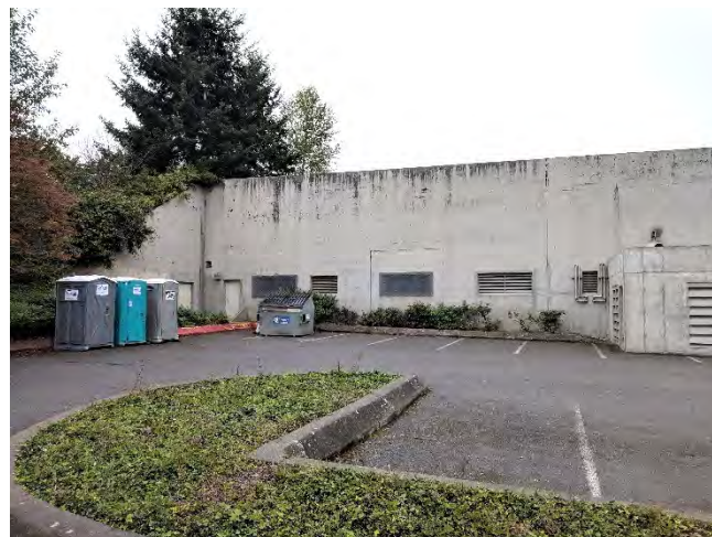
Softening the look of blank walls with green screen vine planting. Also, application of art works effectively to deter tagging.
