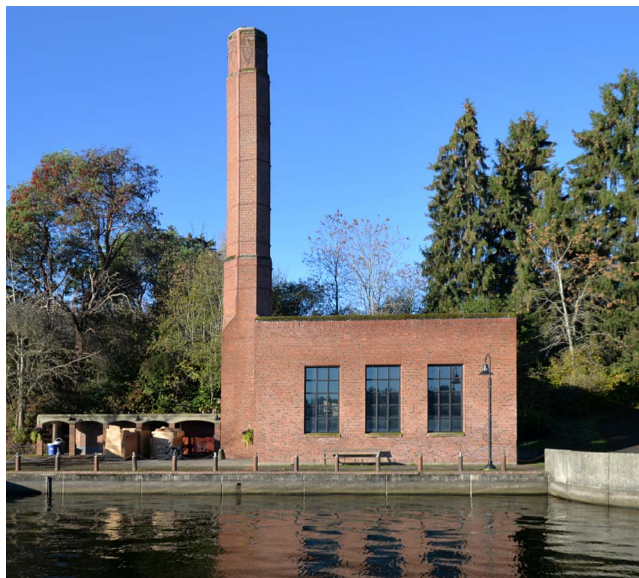
EXISTING BOILER BUILDING & STACK (2) NO SCALE
