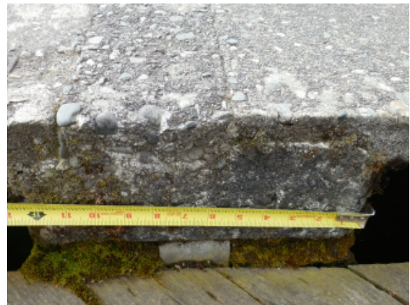
Photo 10A – Pier slab over support
