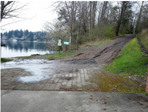
Photo 3A – Gravel maintenance road
