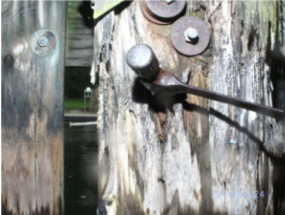
Photo 25C – Decayed pile
