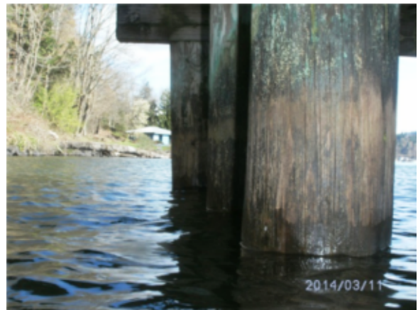
Photo 18B – Treated timber piles
