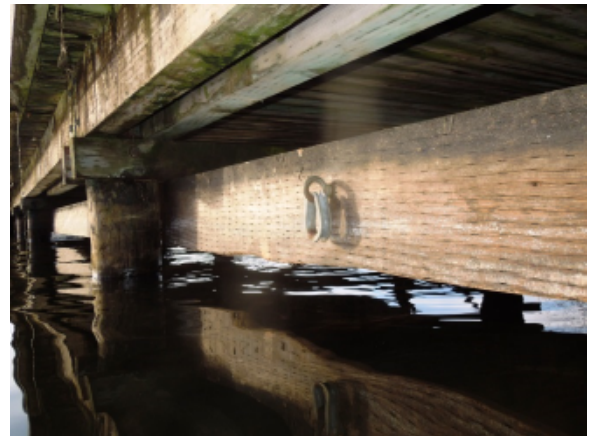
Photo 16B – Typical pier construction
