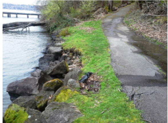
Photo 8B – Rock bulkhead / riprap bank
