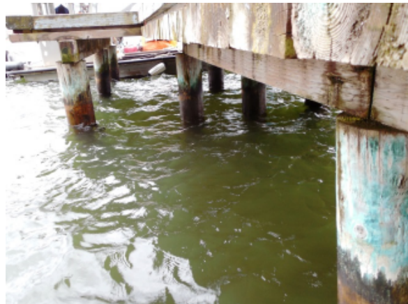
Photo 22B – Looking east along small pier
