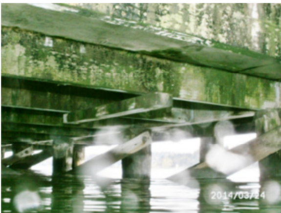
Photo 23C – Large pier substructure
