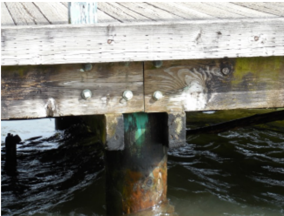
Photo 15B – Typical pier construction
