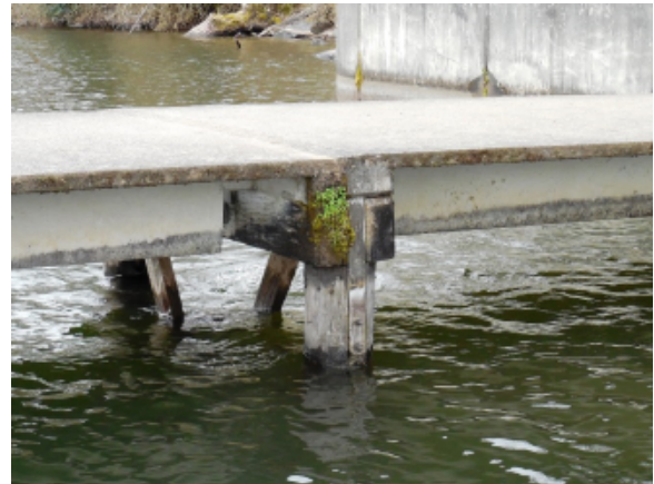
Photo 8A – Typical pier construction
