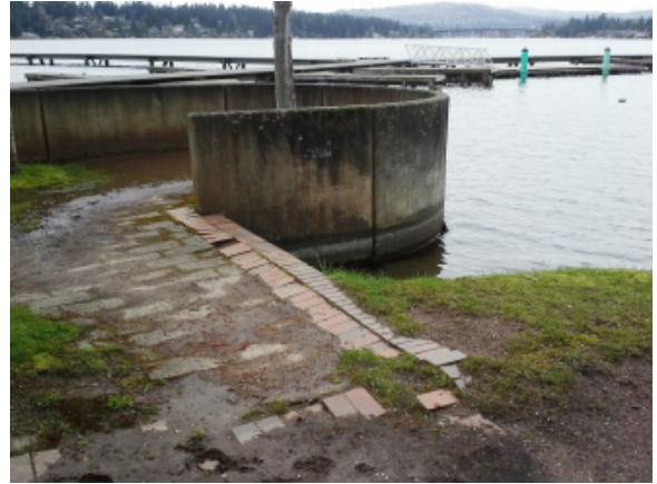
Photo 2A – Brickwork adjacent to bulkhead
