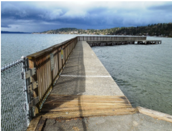
Photo 9C – Large pier, looking north
