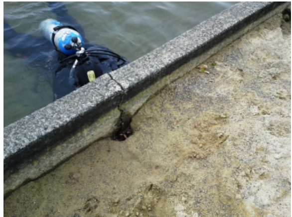
Photo 2C – Cracked bulkhead
