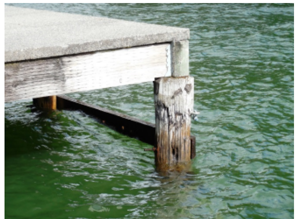
Photo 18C – Large pier deck, stringers and pile
