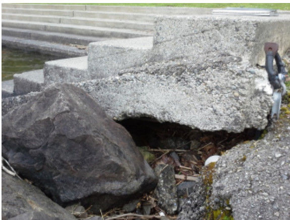
Photo 5B – Shoreline steps
