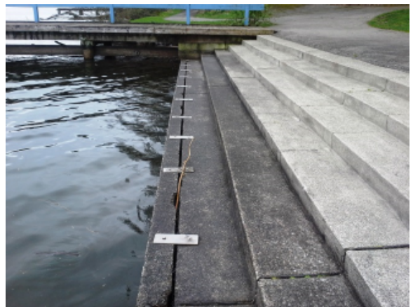
Photo 6B – Shoreline steps / added sheet piling
