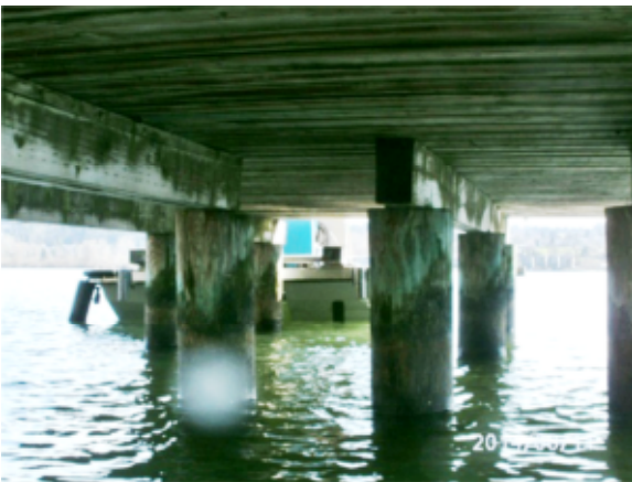
Photo 17B – Treated timber piles
