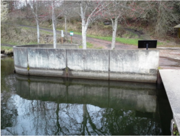
Photo 1A – Concrete bulkhead
