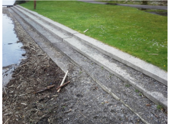
Photo 2B – Shoreline steps
