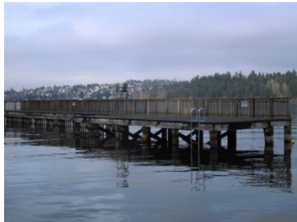
Photo 10C – Large pier, looking south
