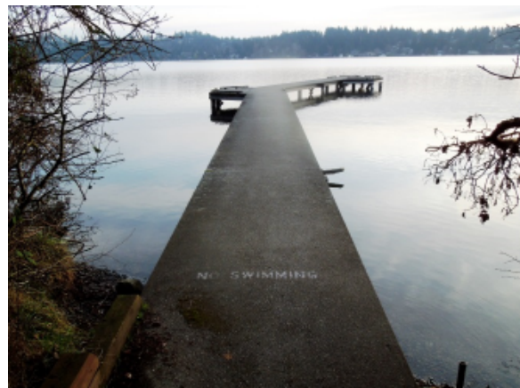
Photo 22A – Small pier
