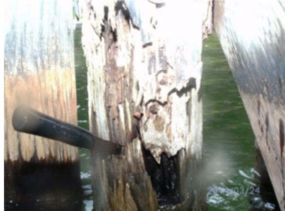
Photo 26C – Decayed pile
