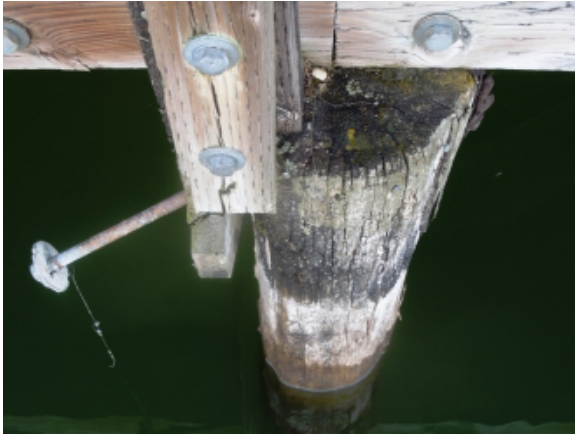
Photo 19C – Loose bracing connector
