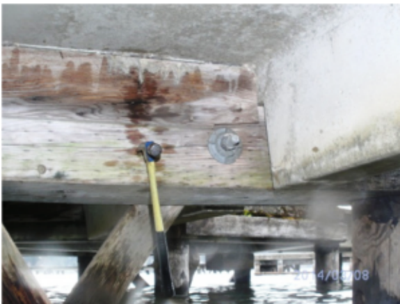
Photo 17A – Precast "T" and timber cap beam
