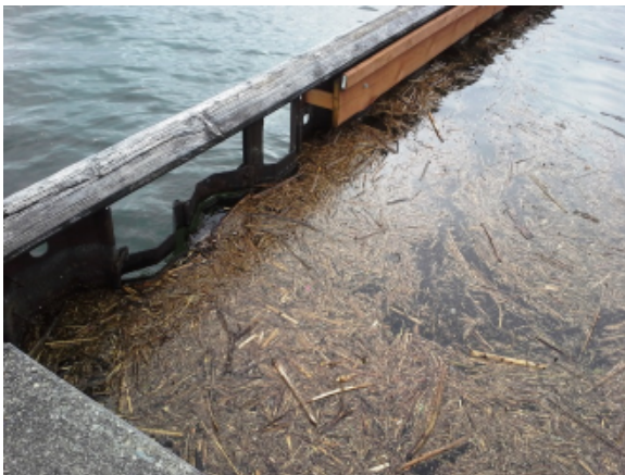
Photo 3B – Sheet piling with fish windows
