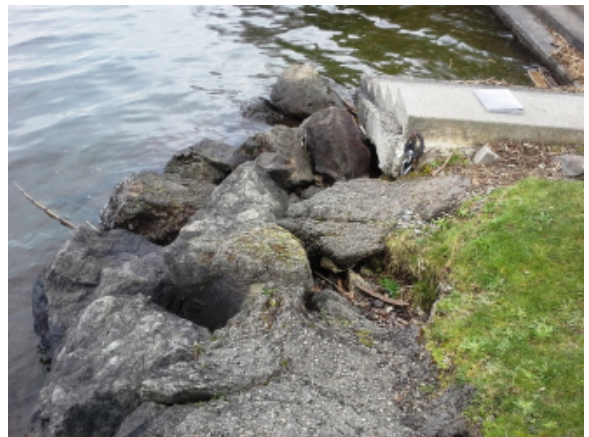
Photo 4B – Rock bulkhead / riprap bank
