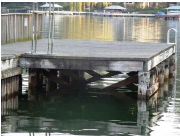
Photo 11C – Large pier, north end
