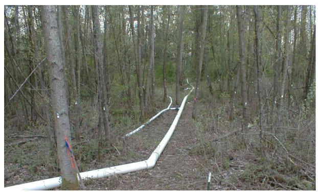
Figure 4.2.15 – Manifold and Braches in a wooded, vegetated sprayfield
