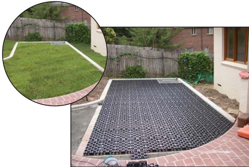
Permeable paving system installed for uncovered parking space. Permeable “grasscrete” paving reduces runoff and contributes to healthy creeks and oceans. (3.4)
