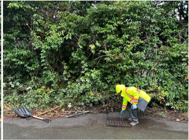
Figure 4. Catch basin after it has been cleared and inspected by CMI staff.
