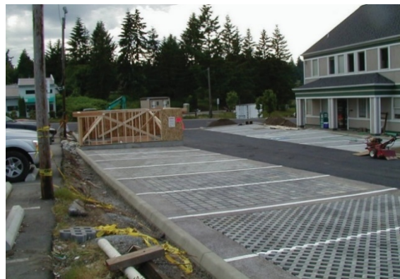
Permeable pavement installation
