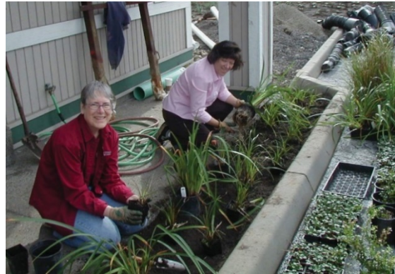
Bioretention during installation
