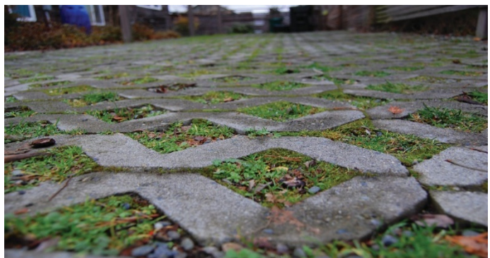
Permeable pavement driveway
