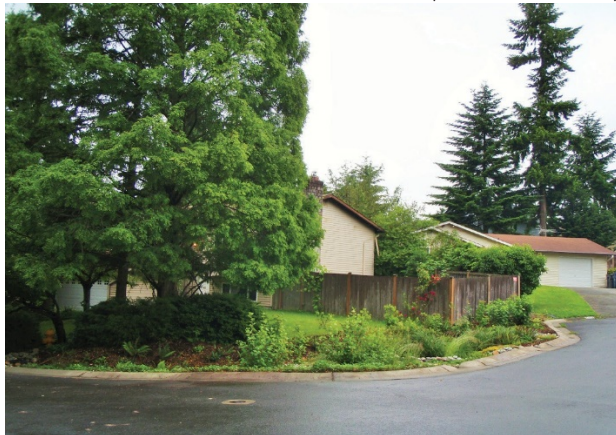
Rain garden collecting road runoff
