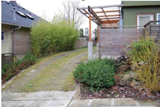
Permeable pavement driveway
