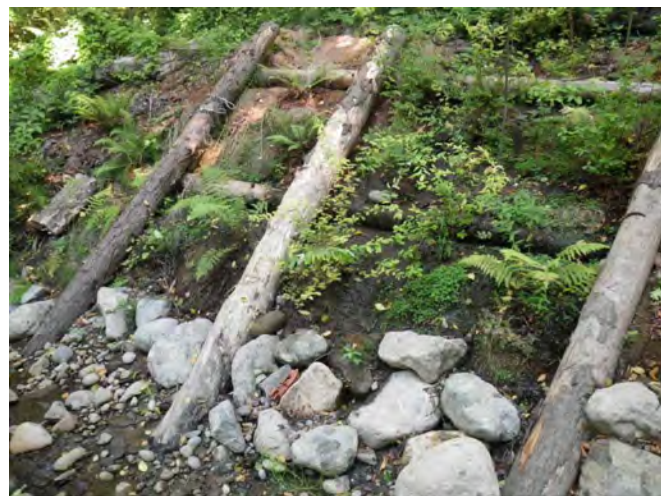
PHOTO EXAMPLE OF FINISHED TIMBER FRAME
