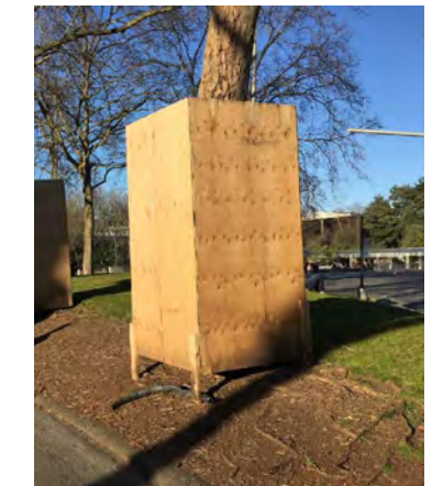
PHOTO EXAMPLE OF SIMILAR TREE PROTECTION DESIGN NOTE: FEET DESIGN IN PHOTO EXAMPLE DIFFERS FROM DETAIL. THIS ALTERNATIVE IS ACCEPTABLE.
