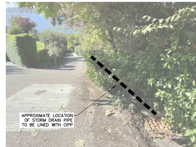
REPAIR PHOTO - FACING SOUTHWEST
