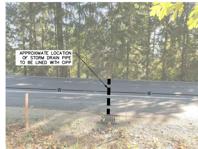
REPAIR PHOTO - FACING SOUTHEAST
