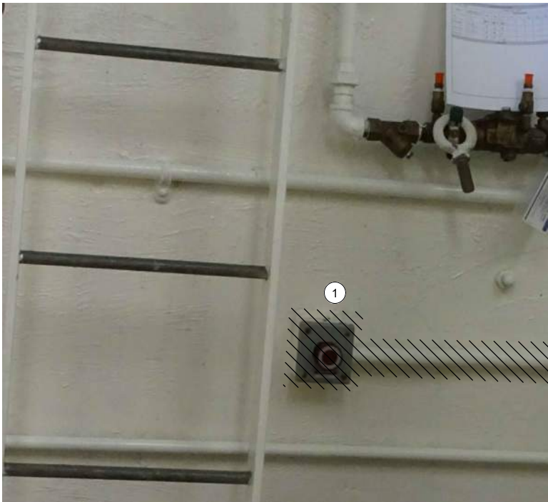
OPERATOR IN TROUBLE PUSHBUTTON AT GRATING LEVEL
