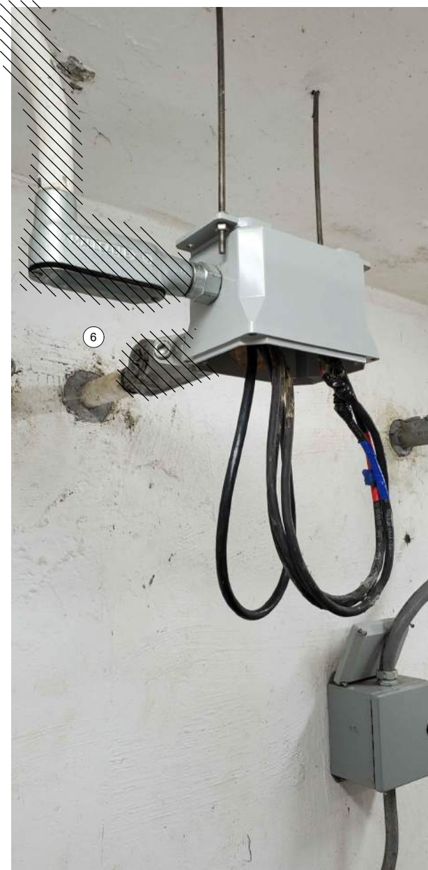
FOGROD LEVEL SENSOR JUNCTION BOX PHOTO C SCALE: NONE
