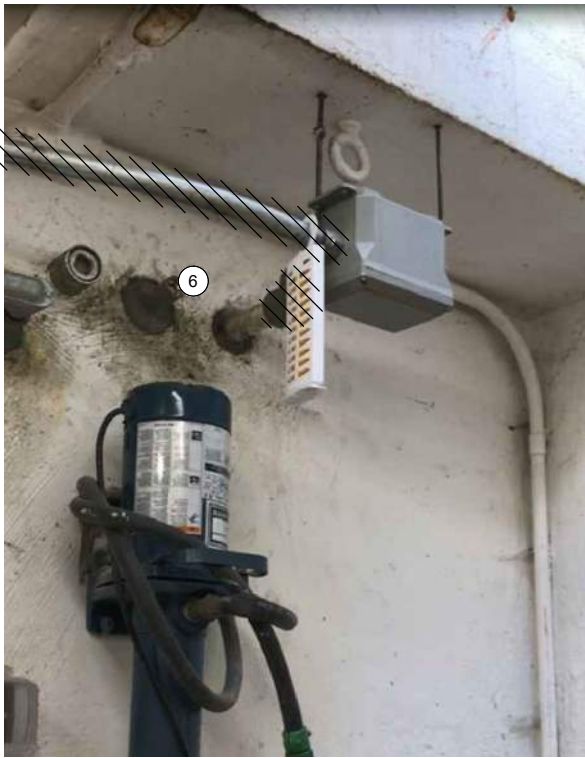
LEVEL FLOAT SWITCHES JUNCTION BOX
