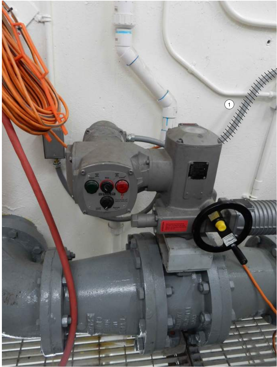
FLUSH VALVE ACTUATOR
