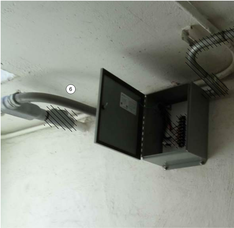
LEVEL FLOAT SWITCHES JUNCTION BOX
