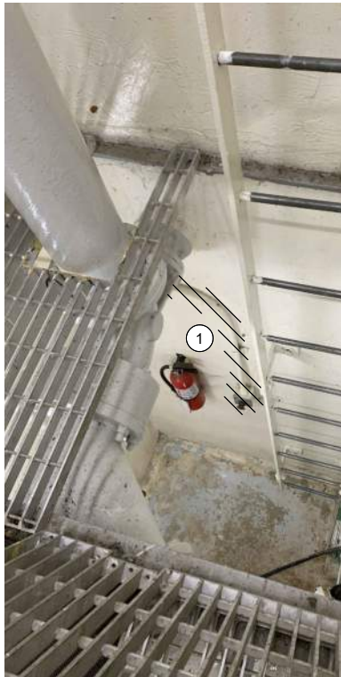
OPERATOR IN TROUBLE PUSHBUTTON AT PUMP LEVEL
