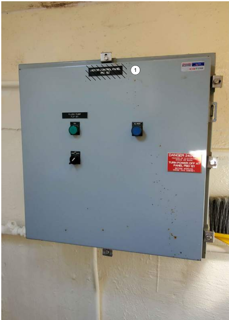
MOTOR CONTROL PANEL EXTERIOR
