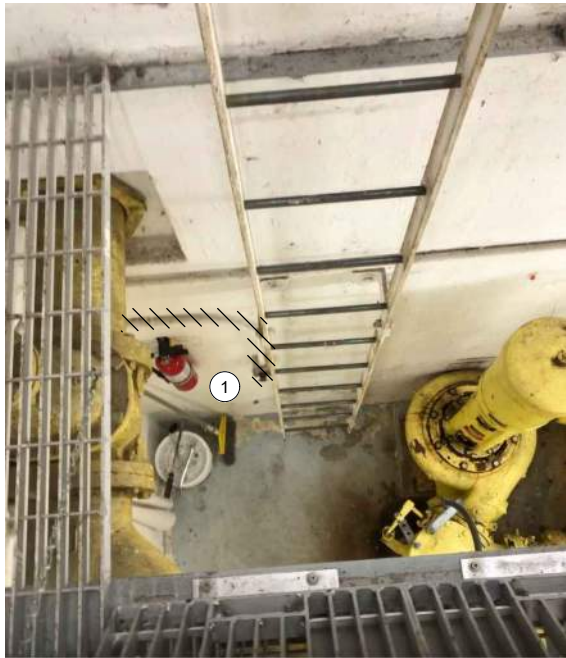
OPERATOR IN TROUBLE PUSHBUTTON AT PUMP LEVEL
