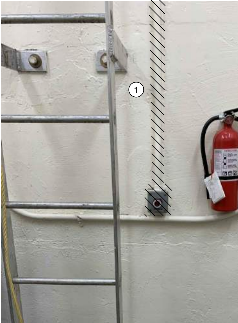
OPERATOR IN TROUBLE PUSHBUTTON AT GRATING LEVEL
