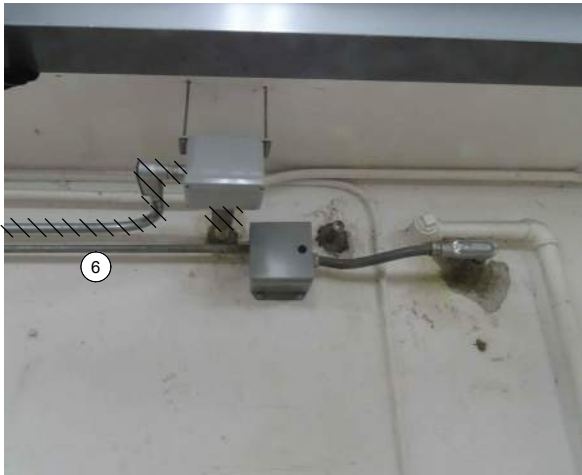
LEVEL FLOAT SWITCHES JUNCTION BOX PHOTO D SCALE: NONE
