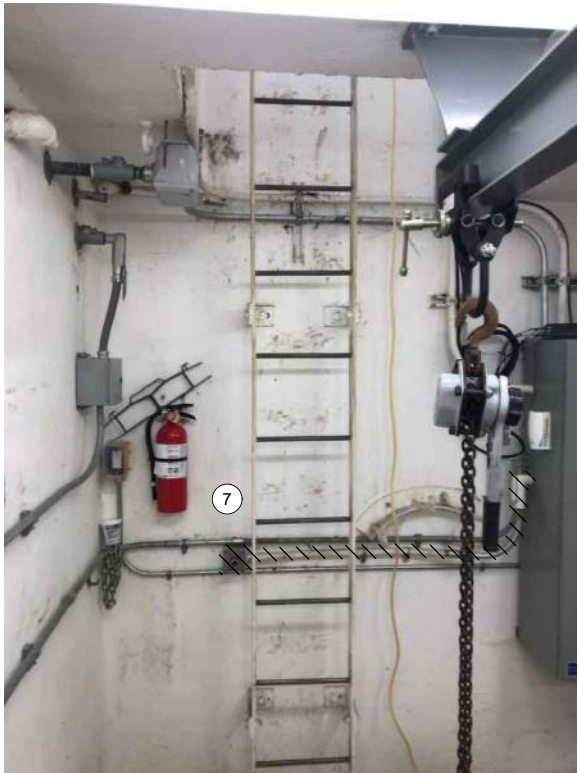
OPERATOR IN TROUBLE PUSHBUTTON AT GRATING LEVEL
