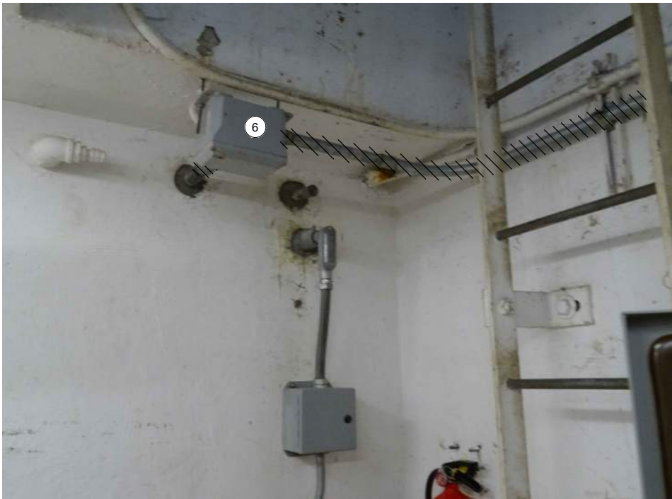
LEVEL FLOAT SWITCHES JUNCTION BOX
