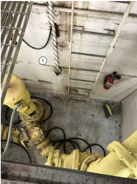
OPERATOR IN TROUBLE PUSHBUTTON AT PUMP LEVEL
