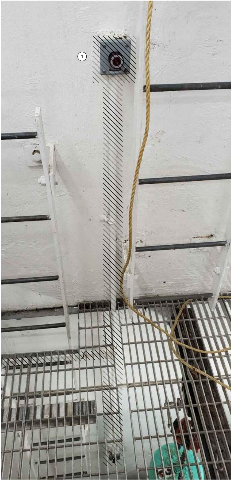
OPERATOR IN TROUBLE PUSHBUTTONS
