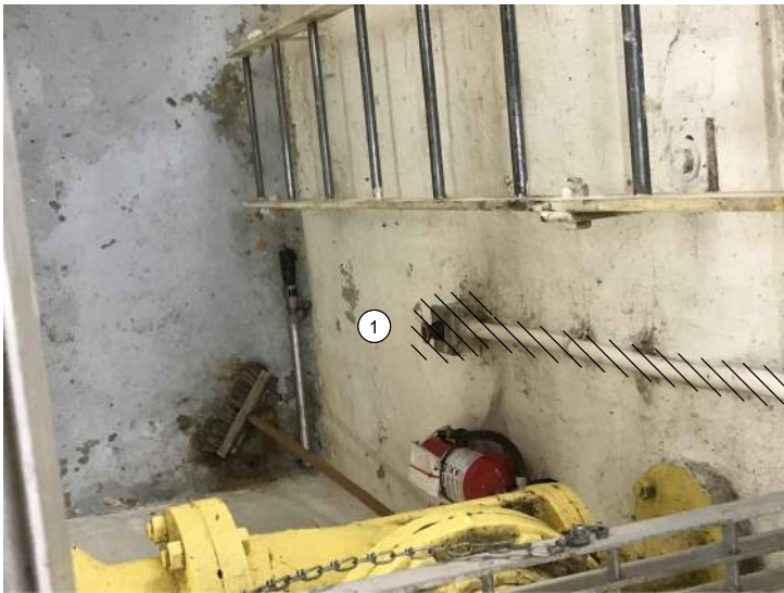
OPERATOR IN TROUBLE PUSHBUTTON AT PUMP LEVEL PHOTO B SCALE: NONE
