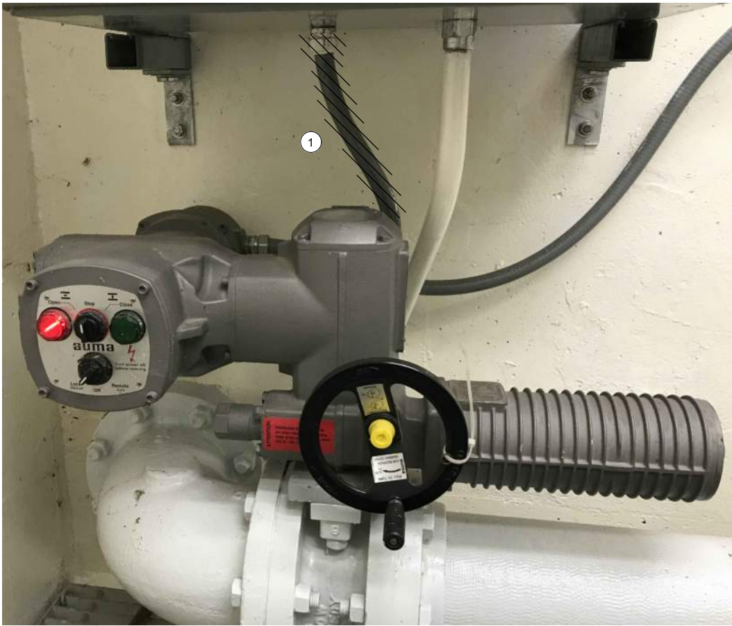
FLUSH VALVE ACTUATOR
