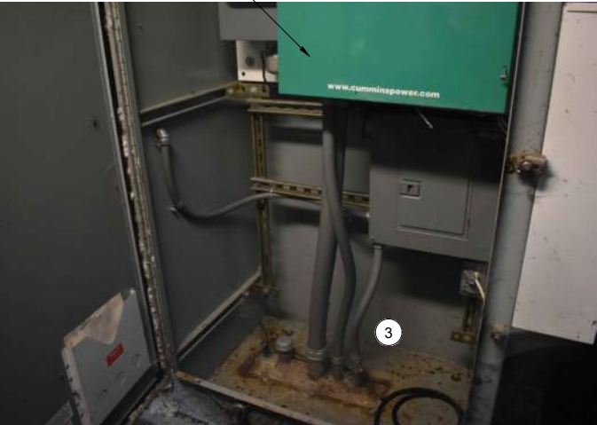
CONDUIT ENTRANCE TO GENERATOR & ATS ENCLOSURE
