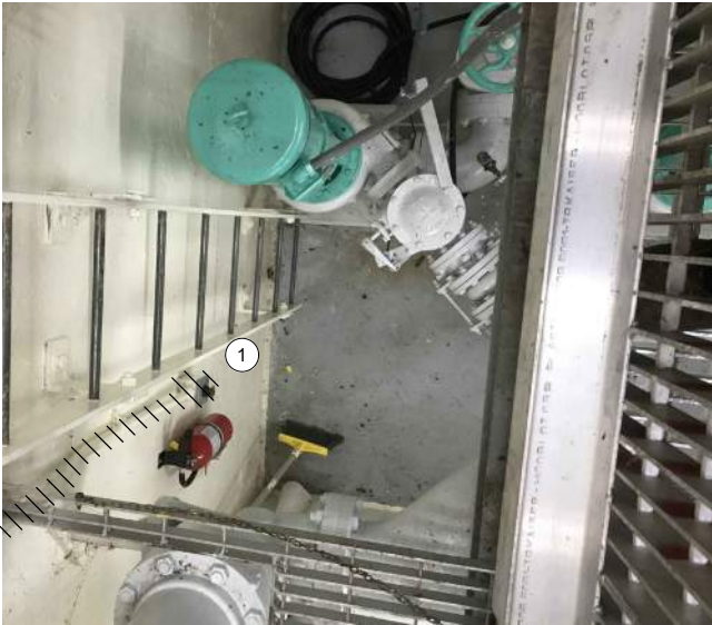
OPERATOR IN TROUBLE PUSHBUTTON AT PUMP LEVEL
