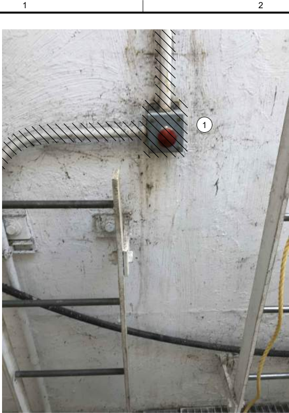
OPERATOR IN TROUBLE PUSHBUTTON AT GRATING LEVEL
