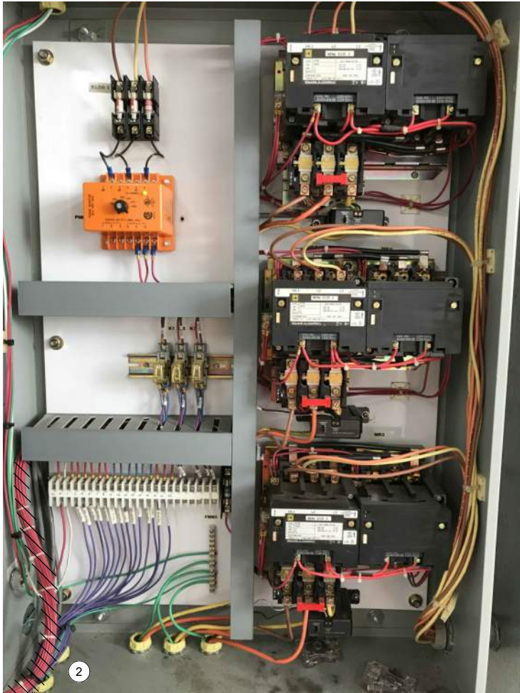
MOTOR CONTROL PANEL INTERIOR BACK PANEL
