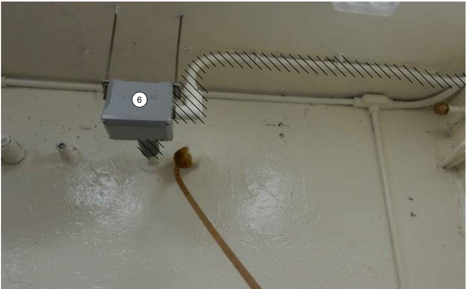
LEVEL FLOAT SWITCHES JUNCTION BOX
