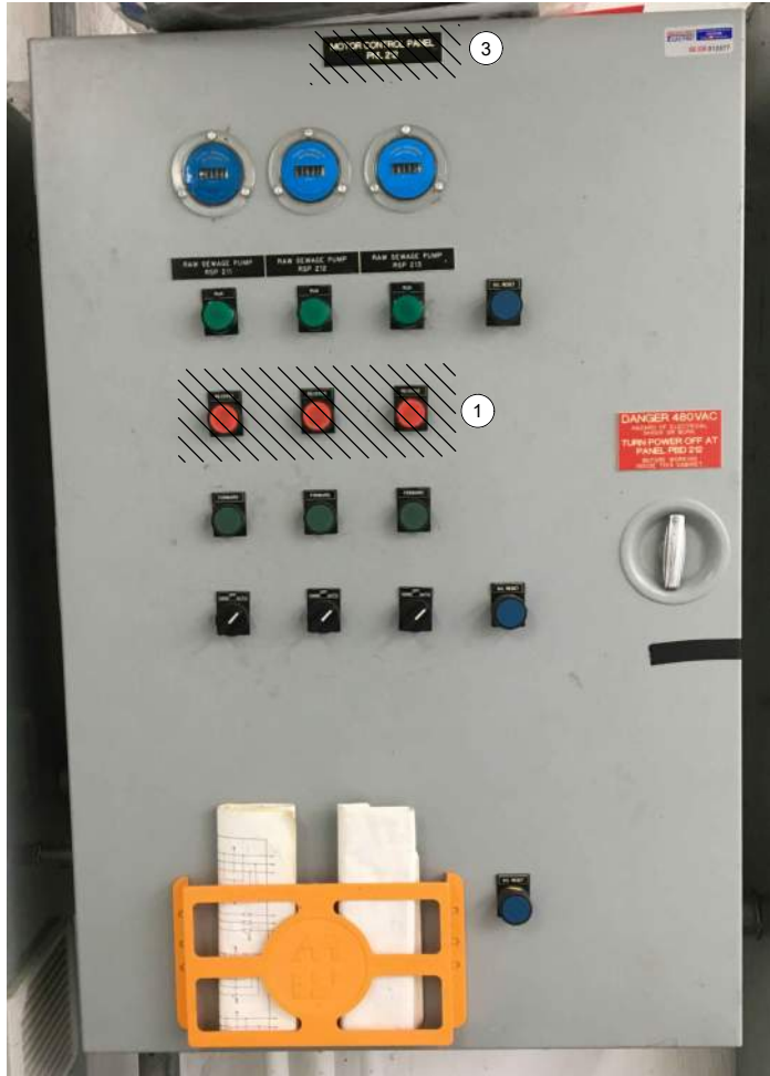
MOTOR CONTROL PANEL EXTERIOR
