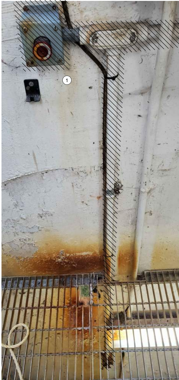
OPERATOR IN TROUBLE PUSHBUTTONS PHOTO A SCALE: NONE
