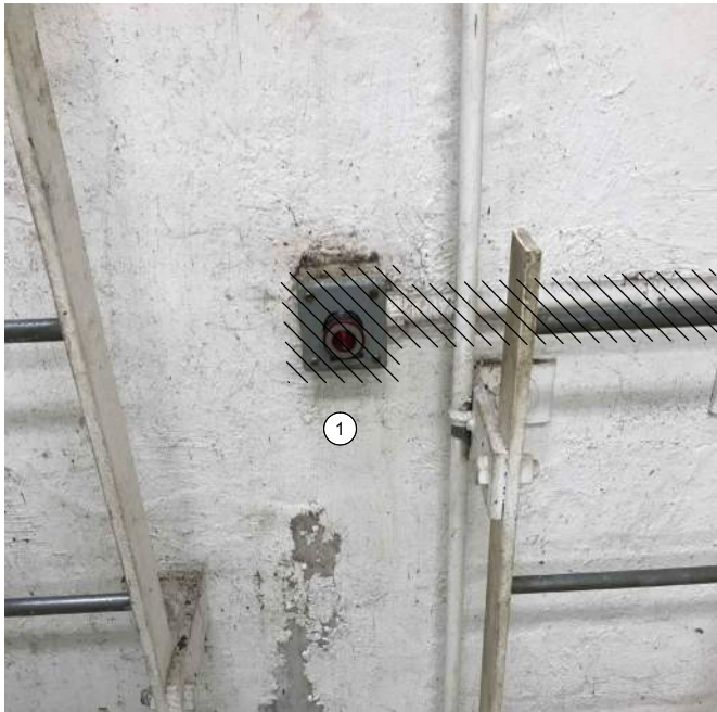
OPERATOR IN TROUBLE PUSHBUTTON AT GRATING LEVEL PHOTO A SCALE: NONE
