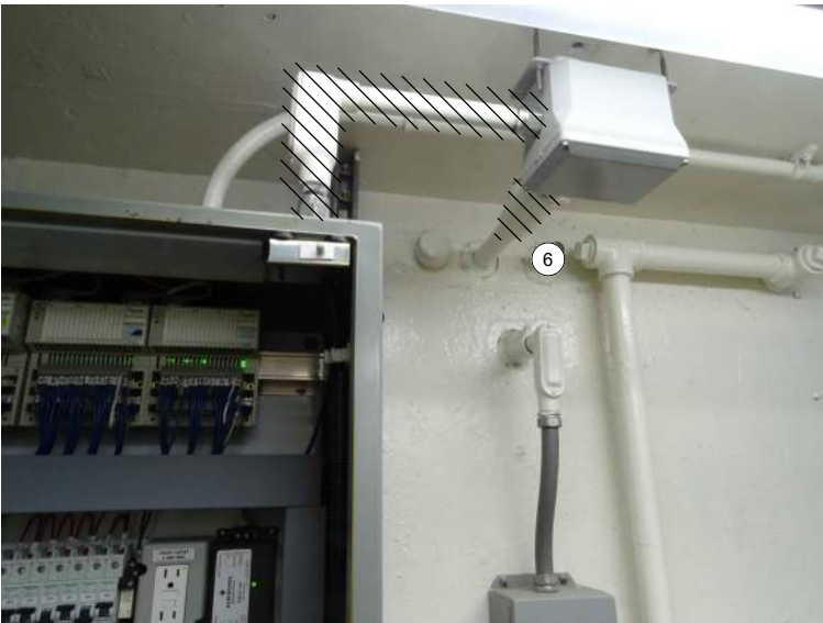
LEVEL FLOAT SWITCHES JUNCTION BOX
