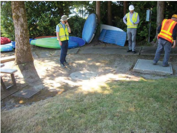
Tree roots appear to be near wetwell which could cause damage
