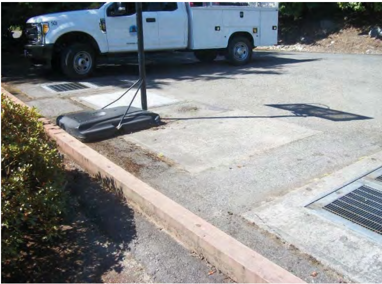
Crews park their trucks in pull off space also used as the vault for below grade generator
