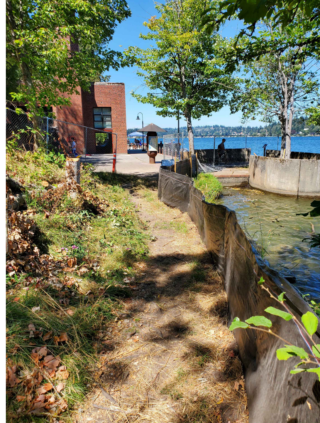
PHOTO 1: CURRENT SILT FENCING NOTE: CHAIN LINK CONSTRUCTION FENCING HAS BEEN REMOVED SINCE THIS PHOTOGRAPH WAS TAKEN
