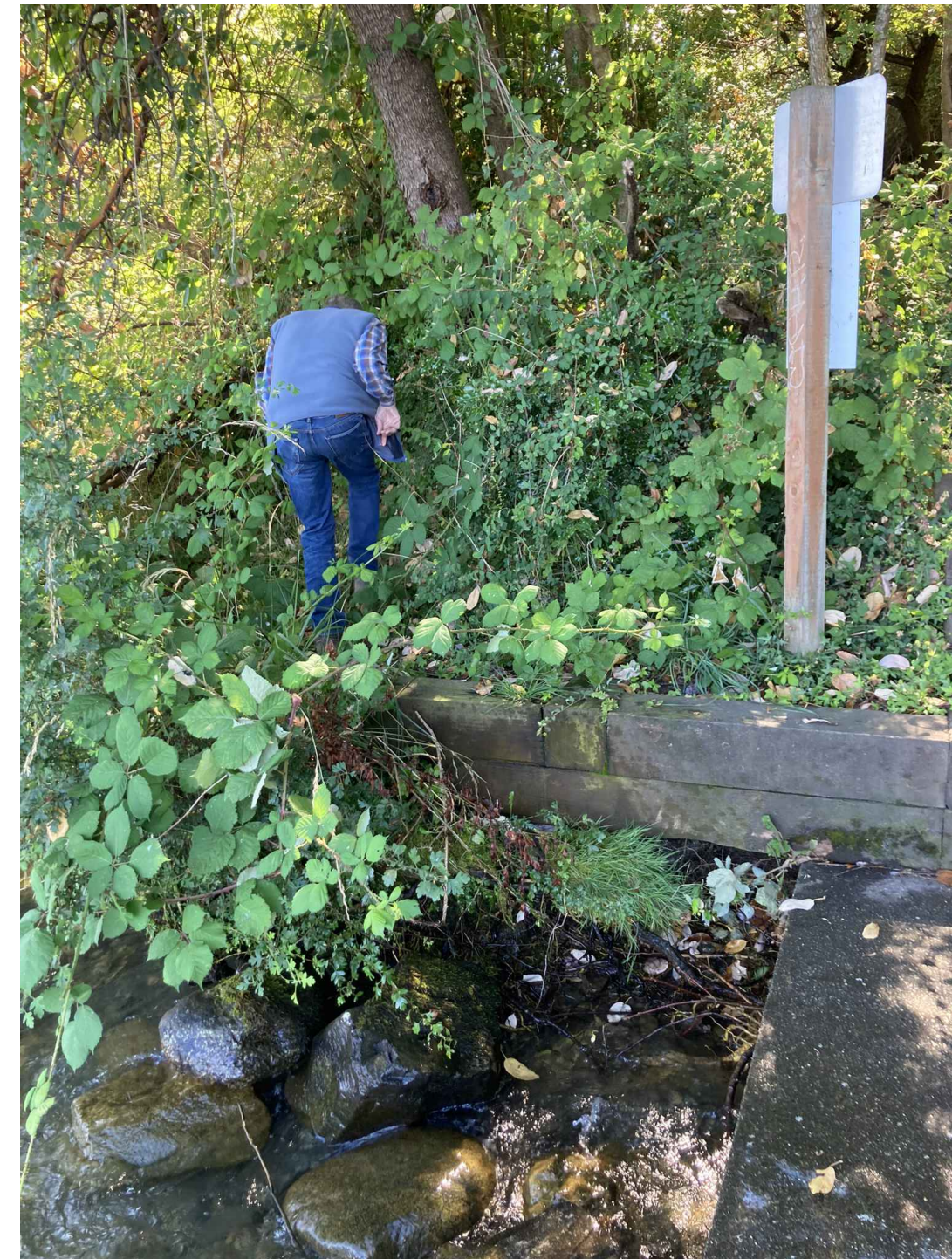
PHOTO 5: TIMBER STEPS VIEW SOUTH
