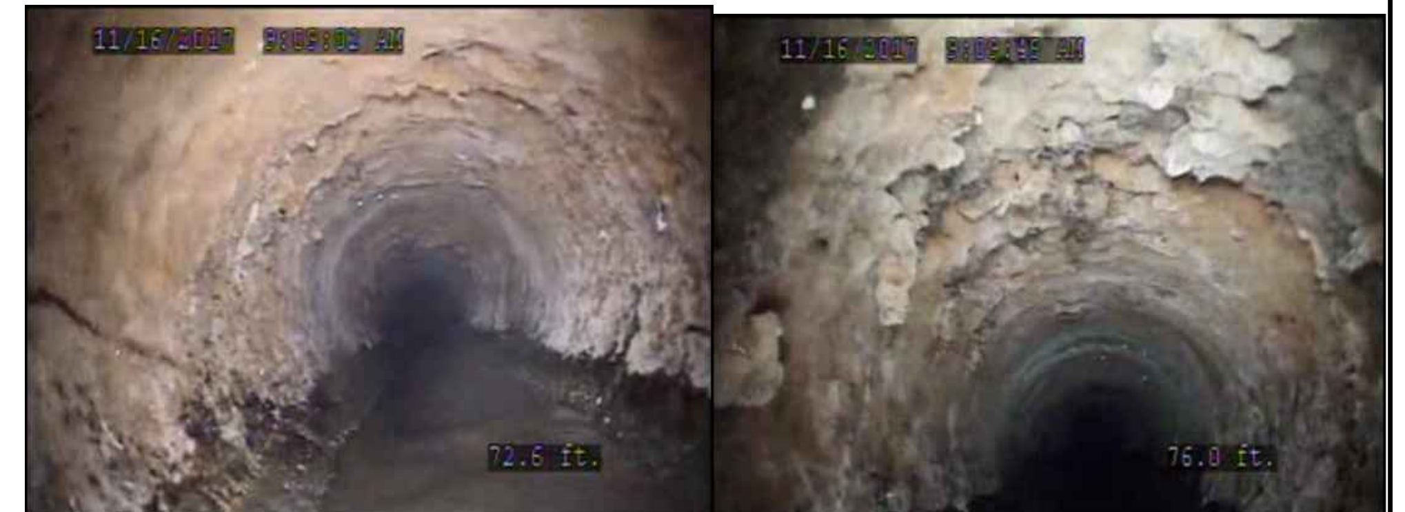
EXISTING MAINLINE CONDITIONS AT SELECT LOCATIONS: MH 68 TO 67
