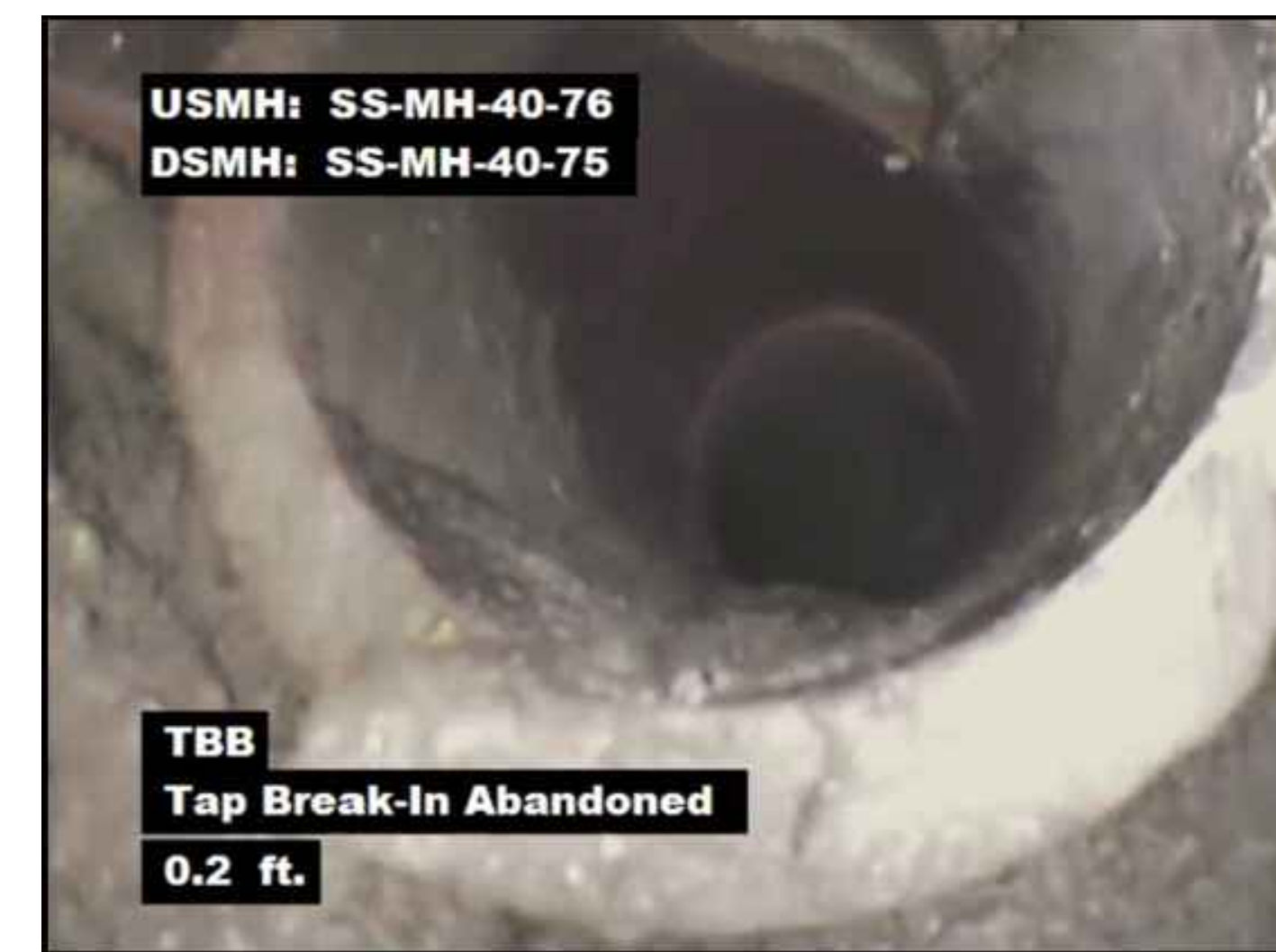
EXISTING LATERAL CONDITIONS AT SELECT LOCATIONS: MH 76 TO MH 75, STA 0+01
