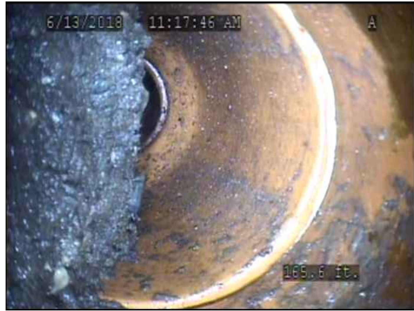
EXISTING LATERAL CONDITIONS AT SELECT LOCATIONS: MH 2.1 TO MH 2.2, STA 1+65
