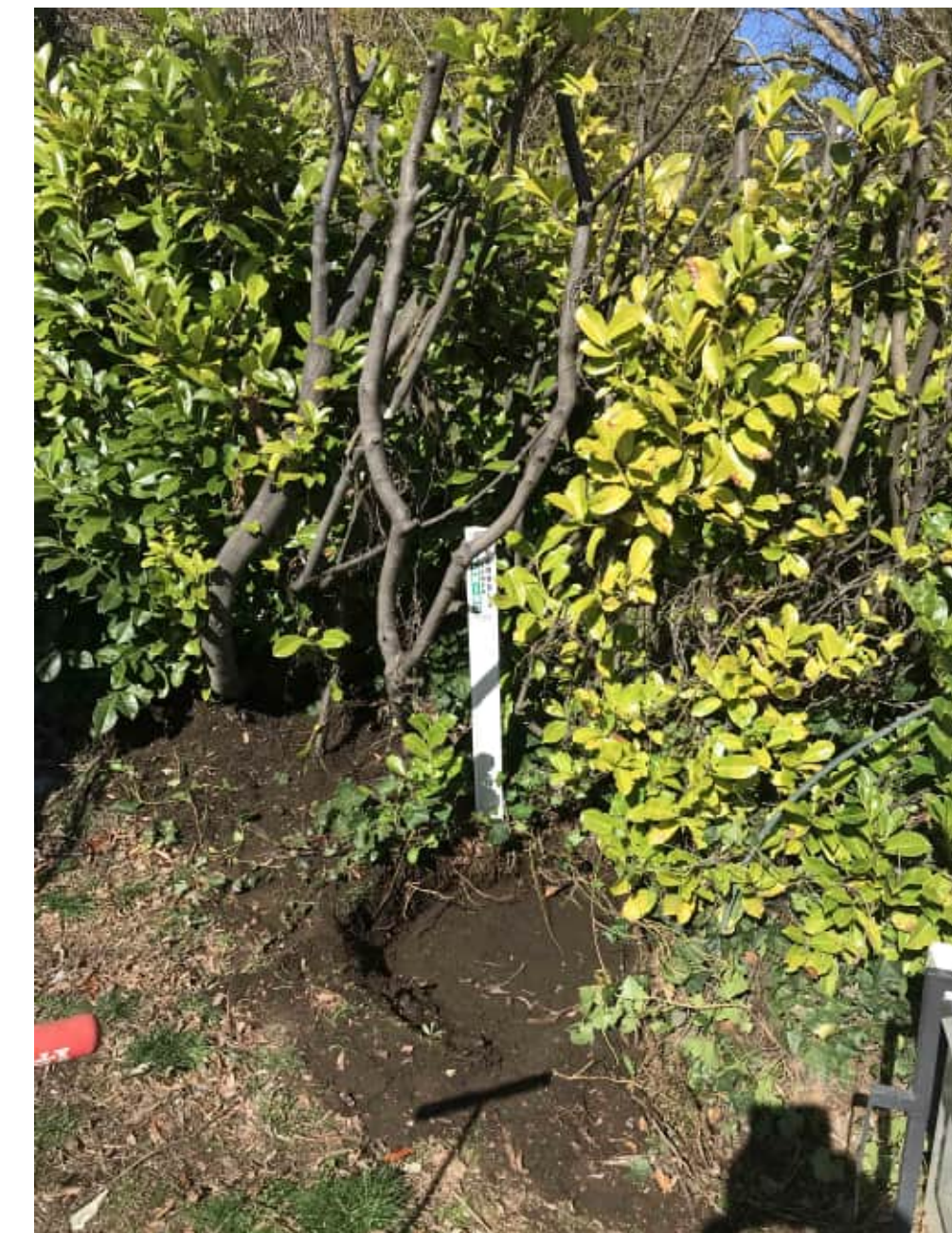
MH LID ACCESS AT SELECT LOCATION: MH 40-2.2
