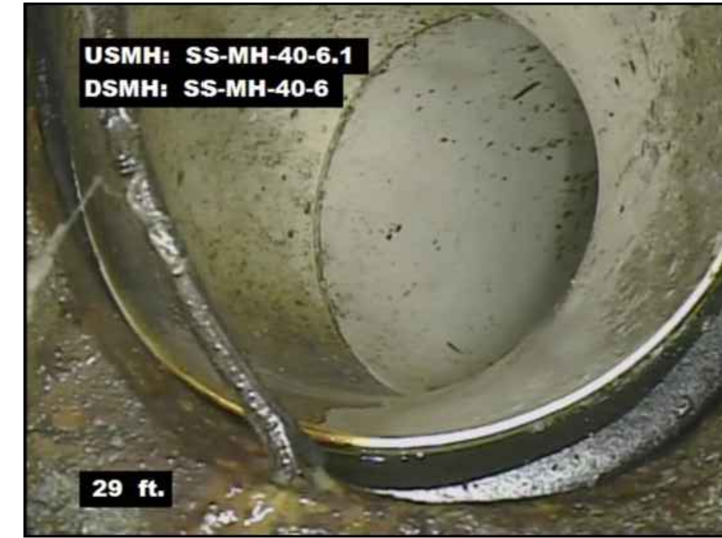
EXISTING LATERAL CONDITIONS AT SELECT LOCATIONS: MH 6.1 TO MH 6, STA 0+29
