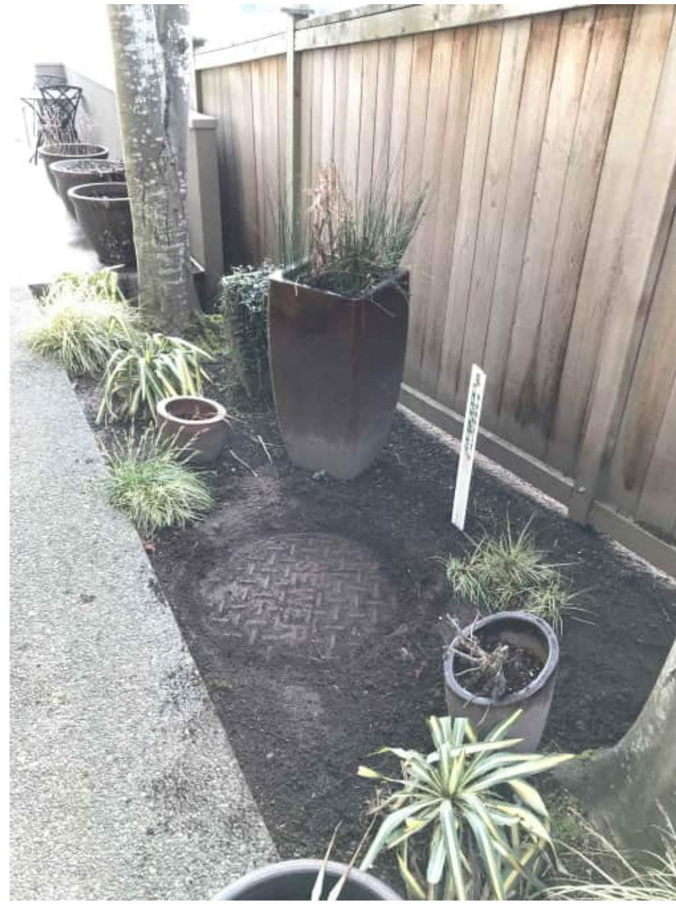
MH LID ACCESS AT SELECT LOCATION: MH 40-950
