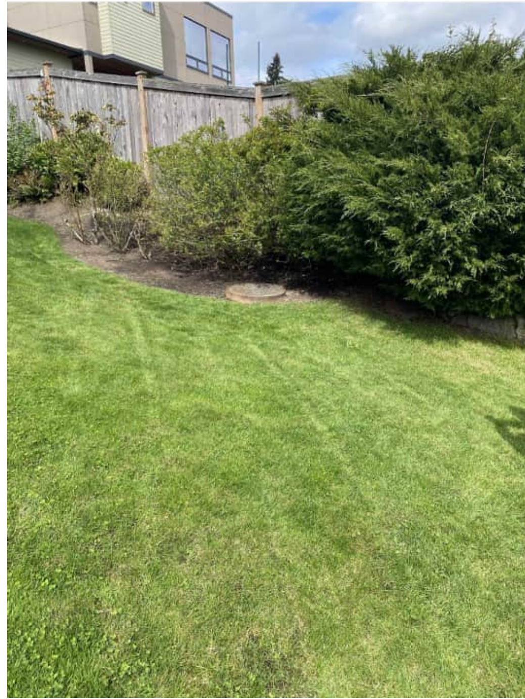
MH LID ACCESS AT SELECT LOCATION: MH 40-47
