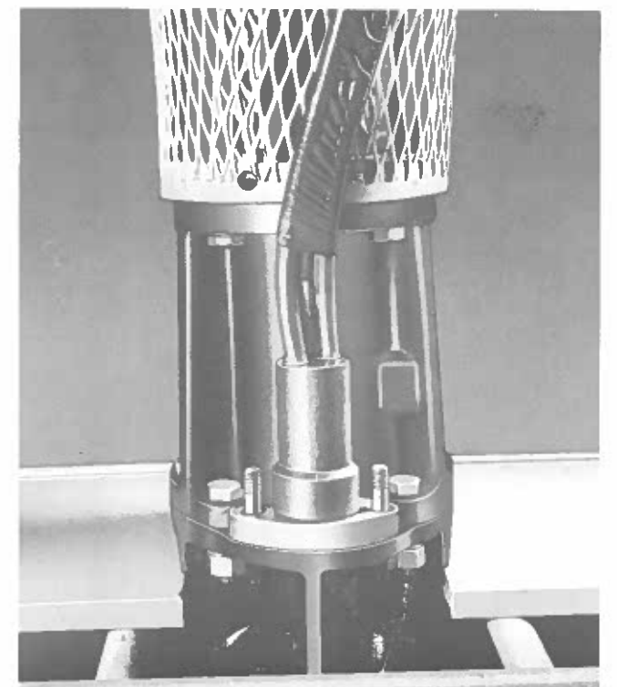
Figure 17 — Terminal Box Installed
