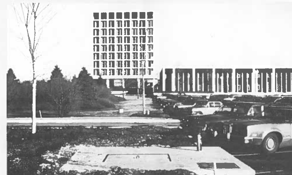
Typical installation of a Byron Jackson submersible pump in an underground vault at the beautiful Allstate Insurance buildings in Northbrook, Illinois.
