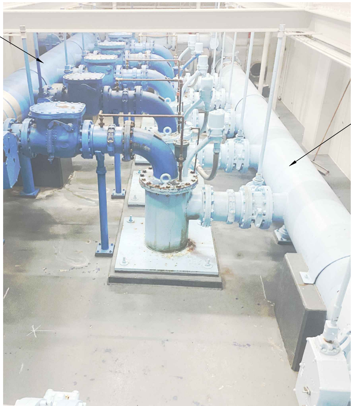
EXISTING PUMP GALLERY
