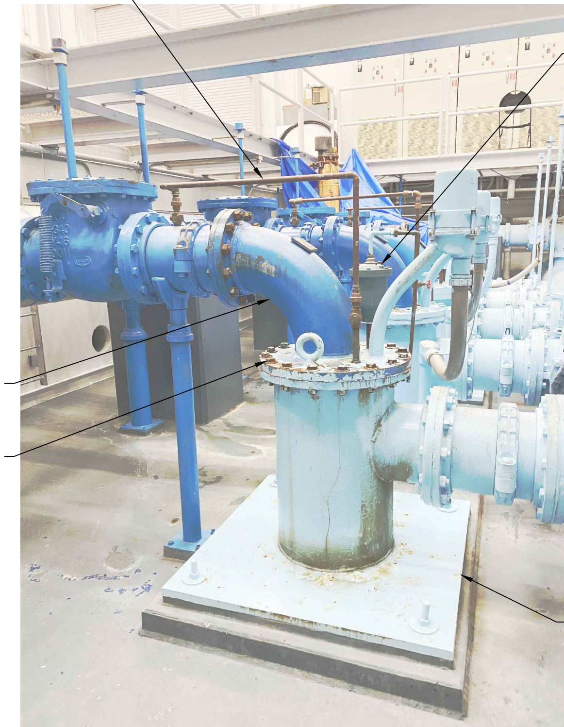
EXISTING PUMP DEMOLITION
