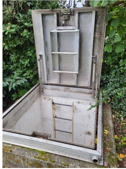
PS 22 lighting and existing dry well grating (left). PS 22 dry well access hatch (right).
