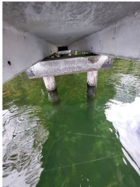
Photo of PS 19 concrete dock under decking.
