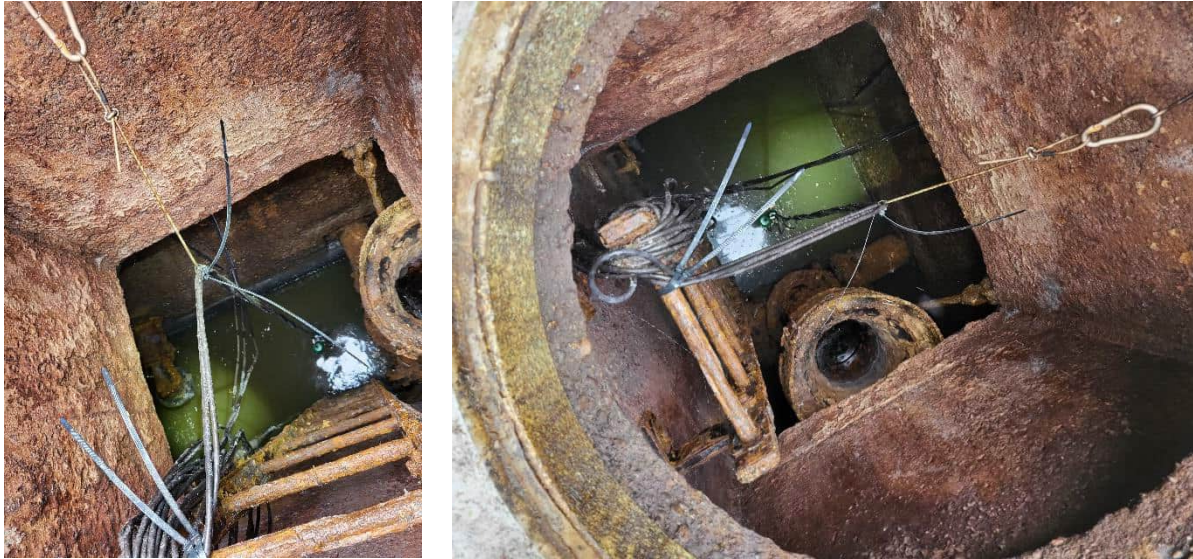
Photos of PS 22 wet well concrete condition.
