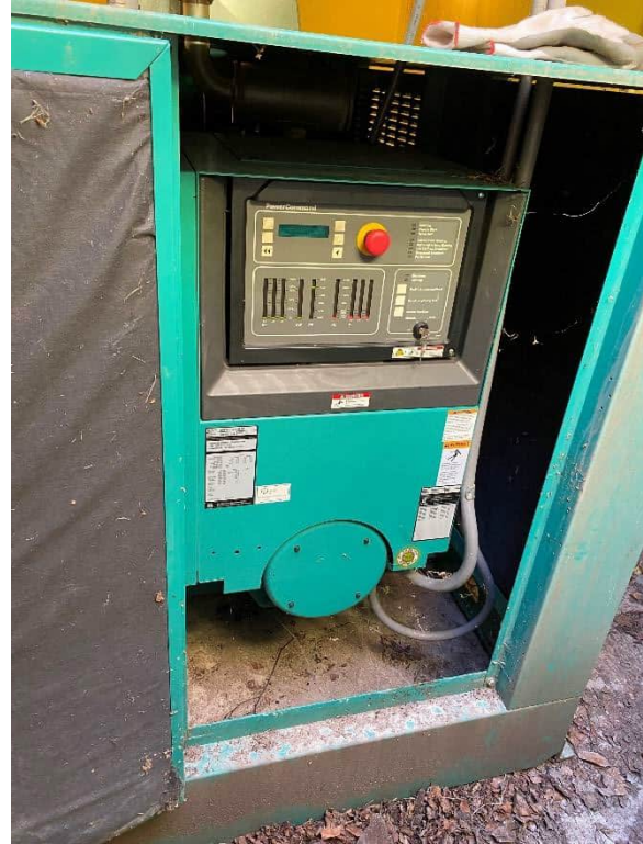
Existing PS 20 dry well grating (left). PS 20 below-grade, on-site diesel generator (right).
