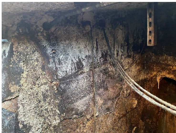
Photos of PS 20 wet well concrete condition and exposed rebar.
