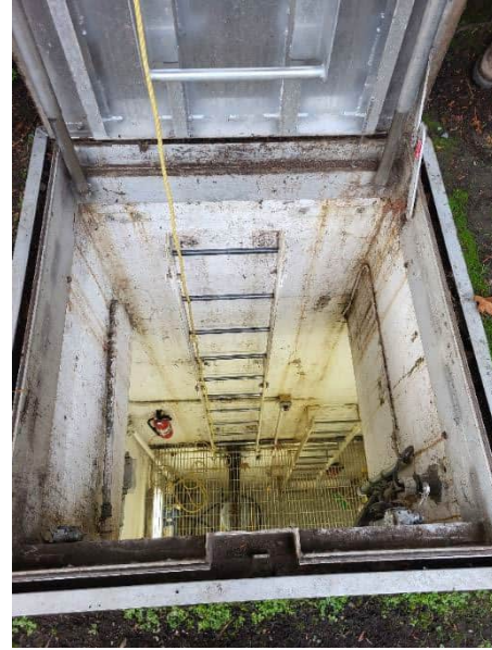
PS 23 lighting in dry well (left). PS 23 dry well access hatch (left).
