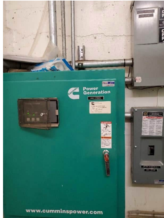
PS 21 upland generator access (left). PS 21 existing Cummins generator ATS (right).
