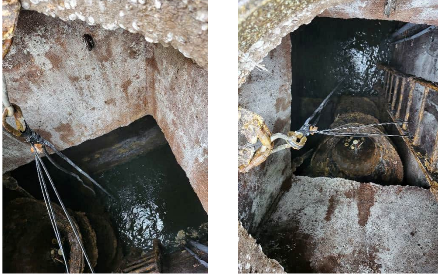
Photos of PS 19 wet well concrete condition.
