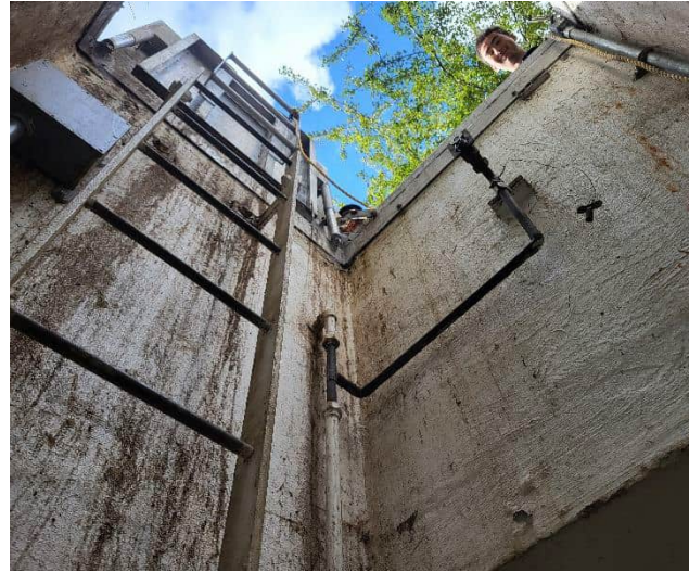
Existing PS 19 grating and ladders in dry well (left). Existing condition of PS 19 dry well entrance (right).
