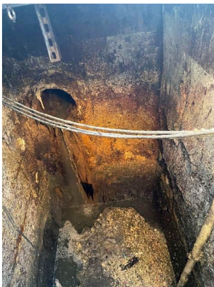
Photos of PS 20 wet well concrete condition and exposed rebar.
