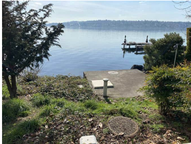
PS 20 site and wet well and dry well access (left).
