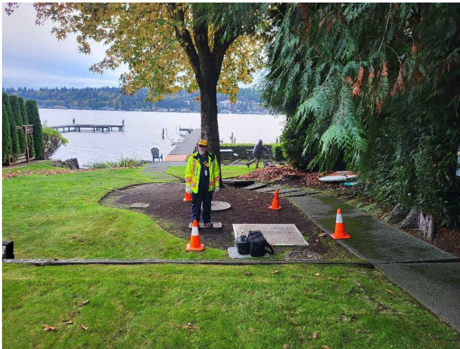
PS 23 wet well and dry well site and access.
