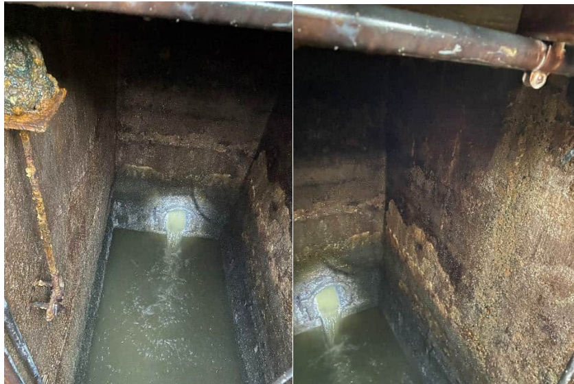
Photos of PS 21 wet well concrete condition.
