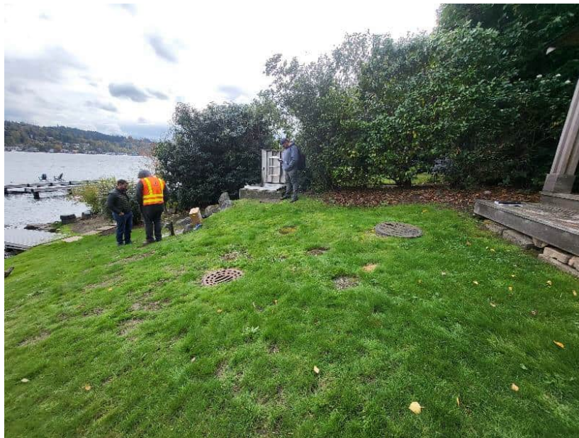
PS 22 site on grassy slope.
