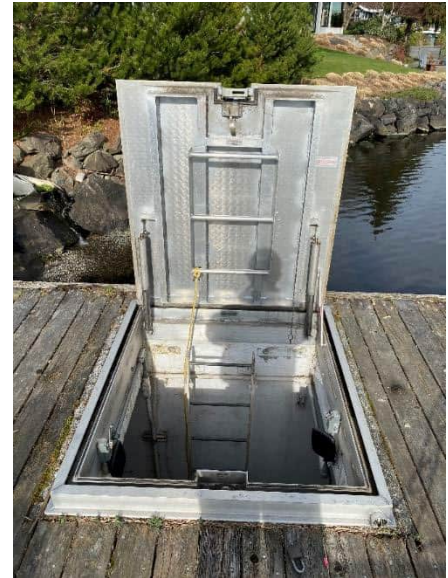
PS 21 dock access from 8002 Avalon Place (left). PS 21 dry well access hatch (right).
