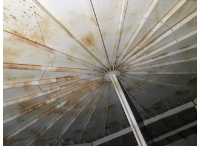
General condition of overhead near center.
