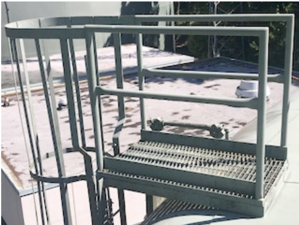
Roof landing – S. reservoir.
