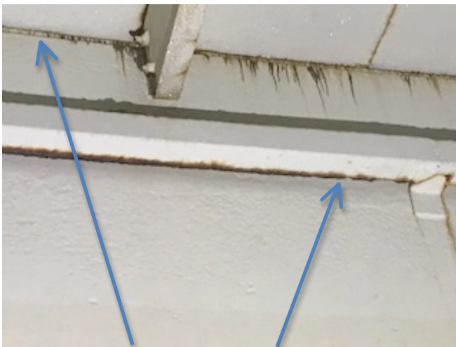
View at “rim angle” and painters rail.
