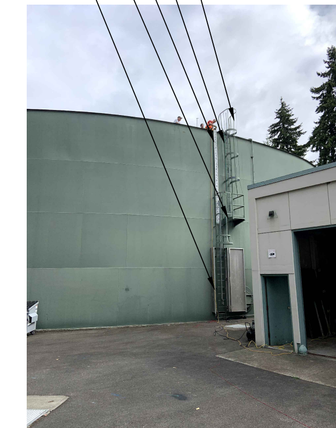
NORTH TANK EXISTING EXTERIOR LADDER, CAGE AND LANDING
