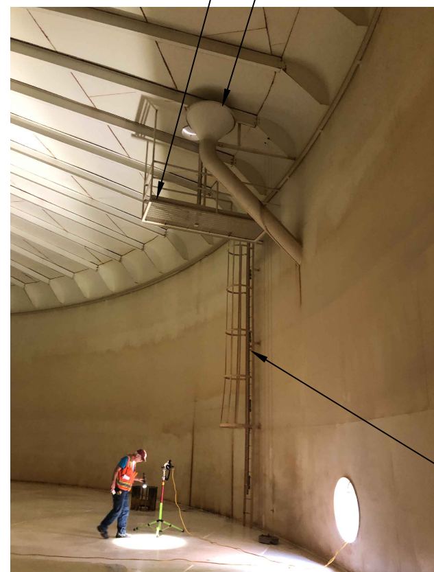
SOUTH TANK EXISTING INTERIOR LADDER
