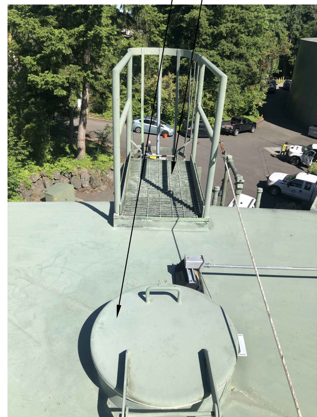
SOUTH TANK EXISTING ACCESS HATCH
