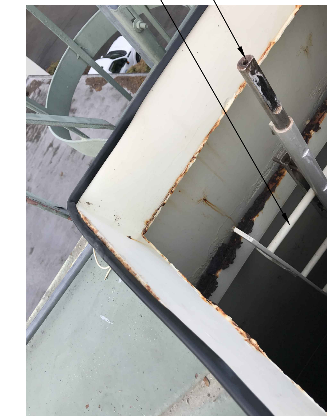
NORTH TANK EXISTING INTERIOR LADDER
