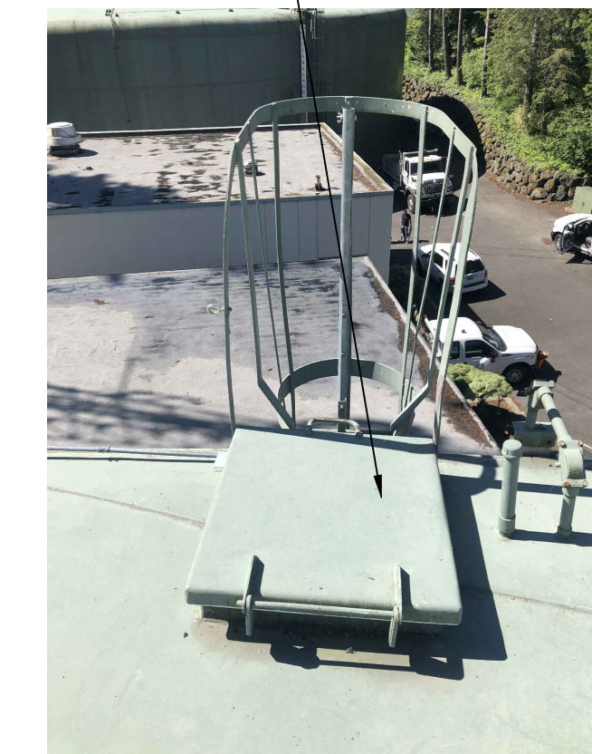
NORTH TANK EXISTING ACCESS HATCH
