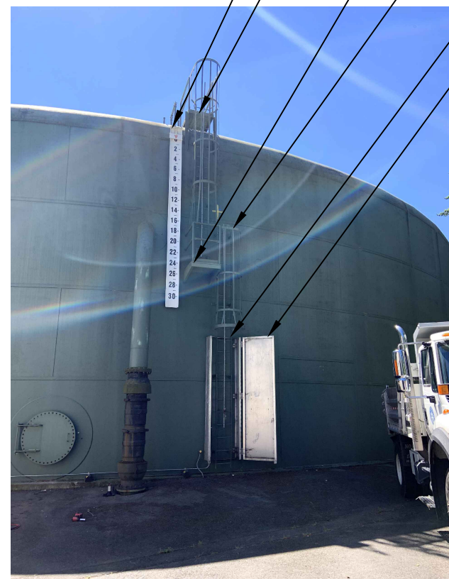
SOUTH TANK EXISTING EXTERIOR LADDER, CAGE AND LANDING
